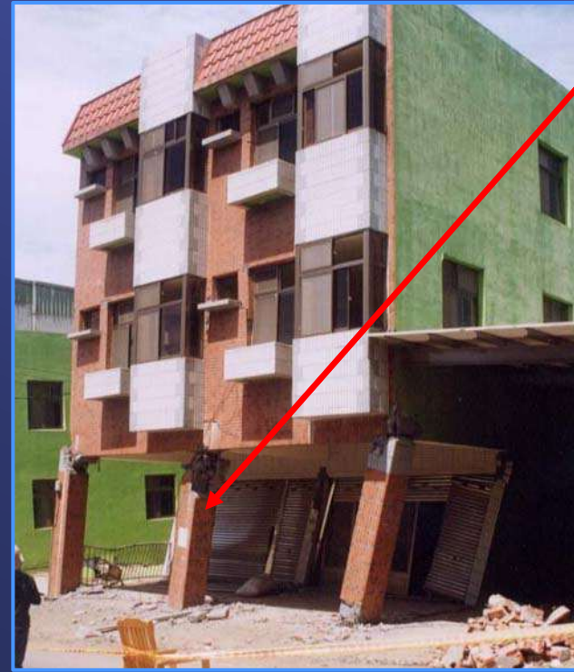
Example of Non-ductile Building
