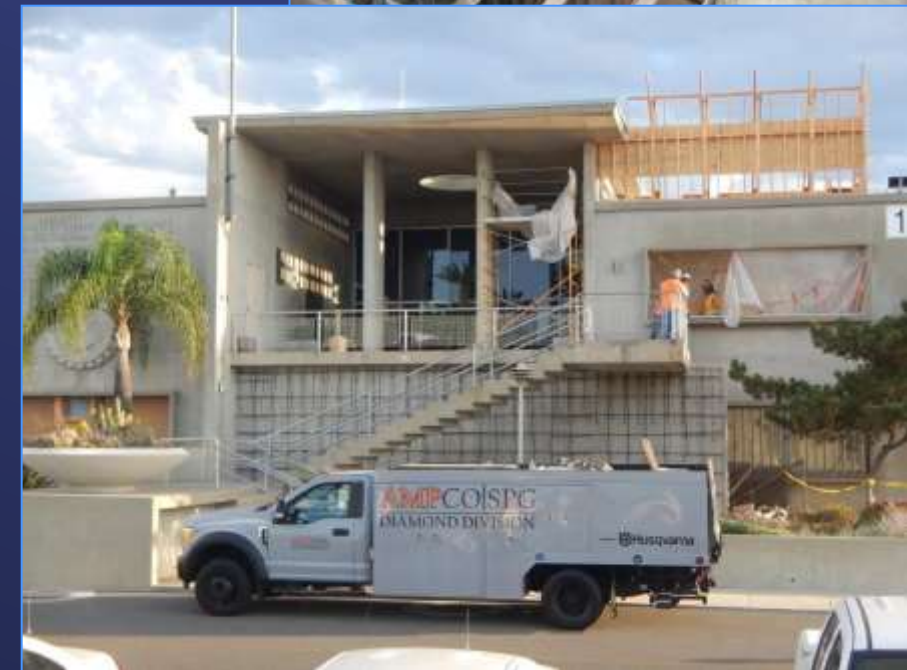
Diemer Admin Building Seismic Upgrade
