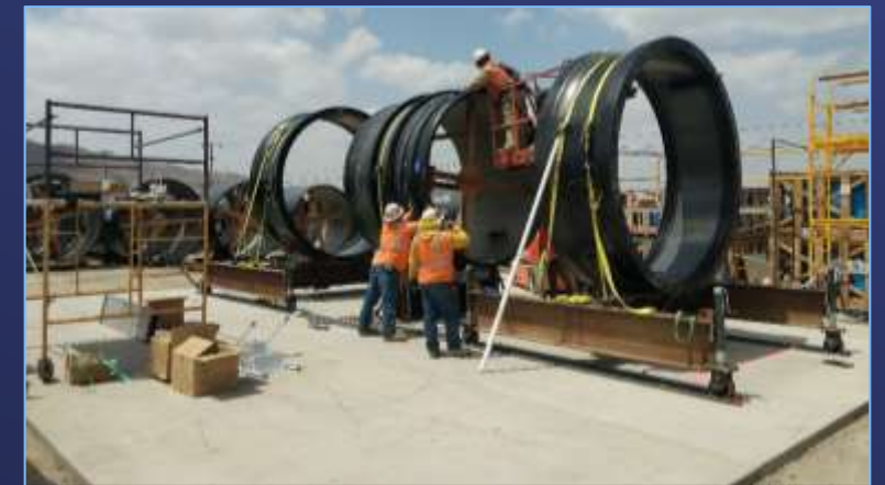
Casa Loma Siphon No.1 – ERDIP Joint Assembly
