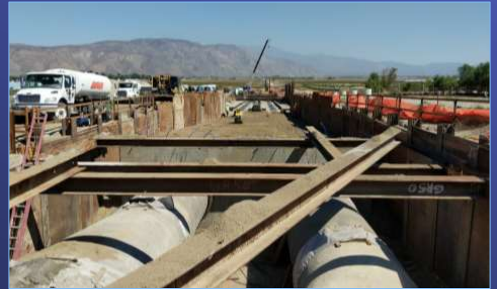
Casa Loma Siphon No. 1 – Excavation (2022)
