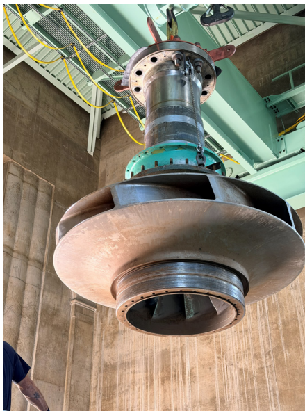
Staff repairing Eagle Unit 1 impeller
