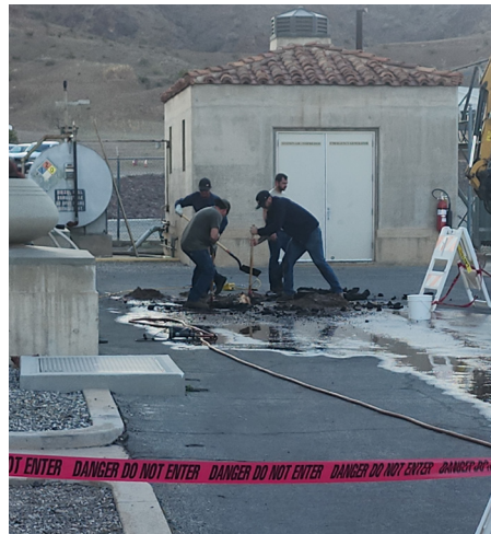
Staff repairing a cooling water leak at Gene pump plant
