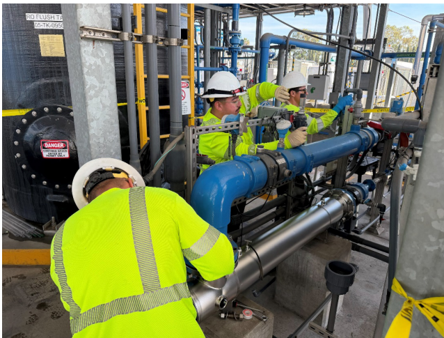
Staff installing UV system effluent pipe (left) and removing RO membrane elements (right) at the PWSC Napolitano Innovation Center demonstration plant
