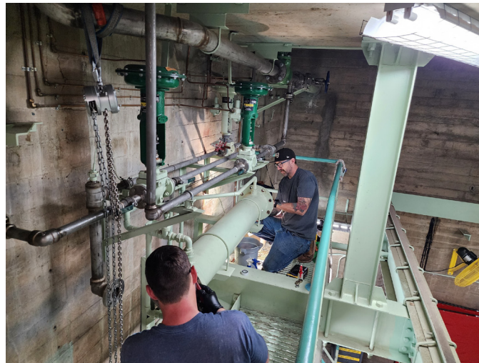
Staff rebuilding Unit 9 bearing heat exchanger at Intake pump plant
