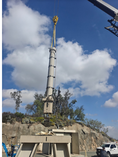
Hydraulic ram and pedestal pictured before removal (left) and staff separating the ram from its pedestal (right)
