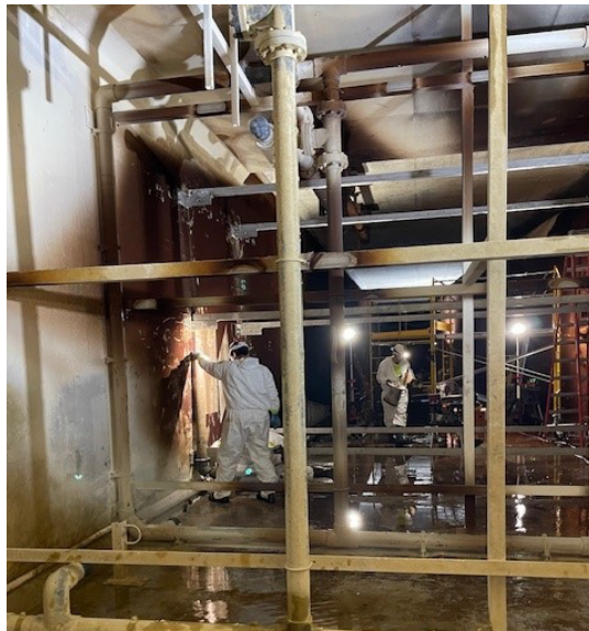
Staff working on new chlorine diffusers at the Diemer plant
