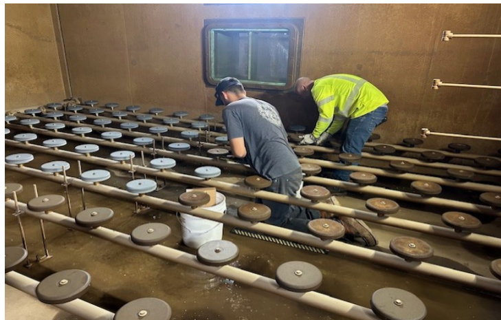
Staff replacing ozone diffuser at Weymouth plant
