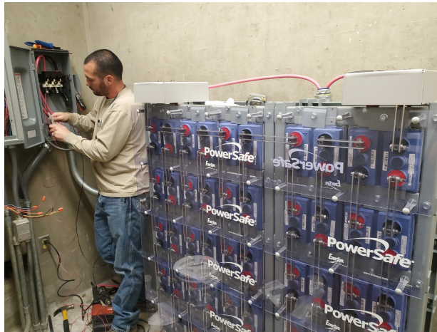
Staff installing new station batteries at Red Mountain Hydroelectric Plant
