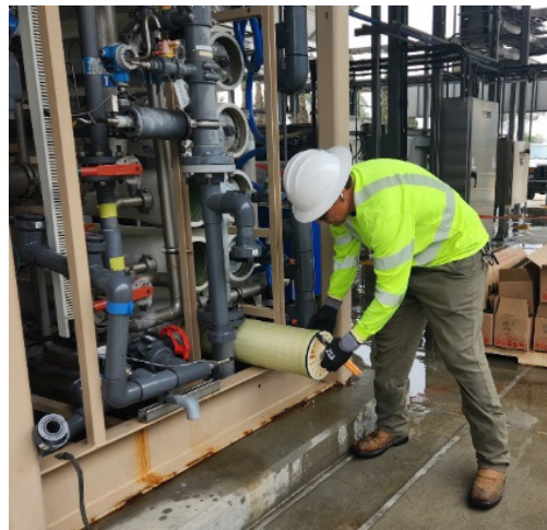
Staff installing UV system effluent pipe (left) and removing RO membrane elements (right) at the PWSC Napolitano Innovation Center demonstration plant
