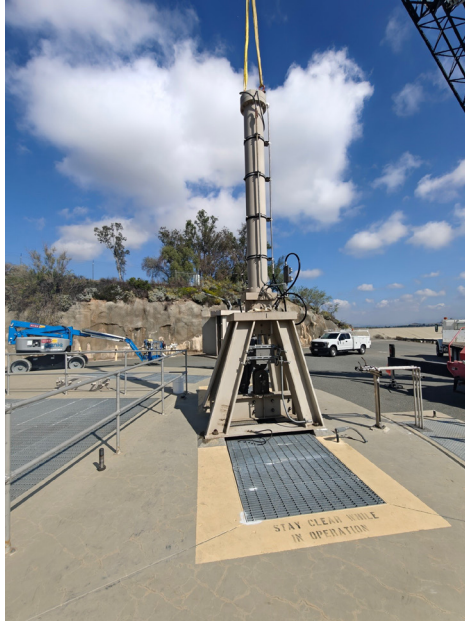
Hydraulic ram and pedestal pictured before removal (left) and staff separating the ram from its pedestal (right)
