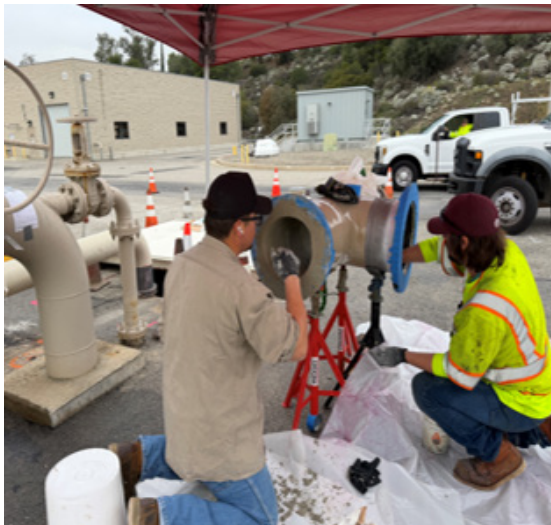
Staff installing a fabricated pipe (left) and the completed installation (right)
