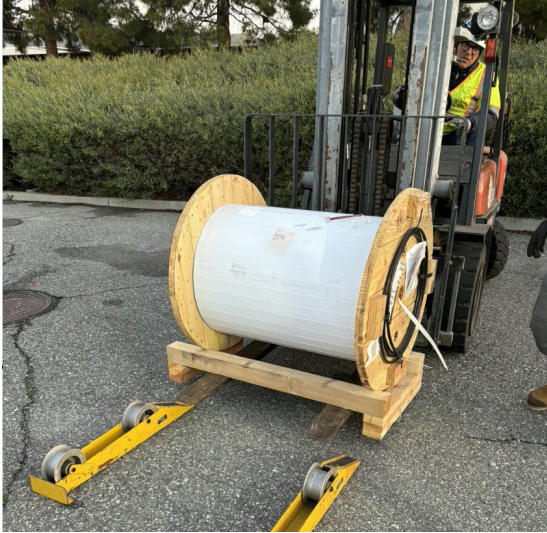
Staging fiber optic cable spool (left) and accessing utility vaults (right) at Weymouth plant
