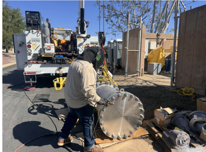
Staff is preparing spools and a valve for installation
