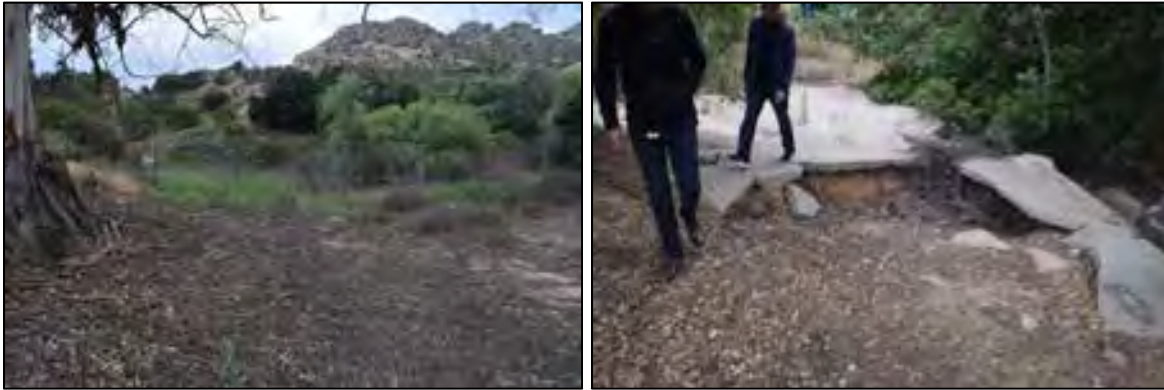
Figure 4 - Earthen Flood Control Basin and Broken Spillway
