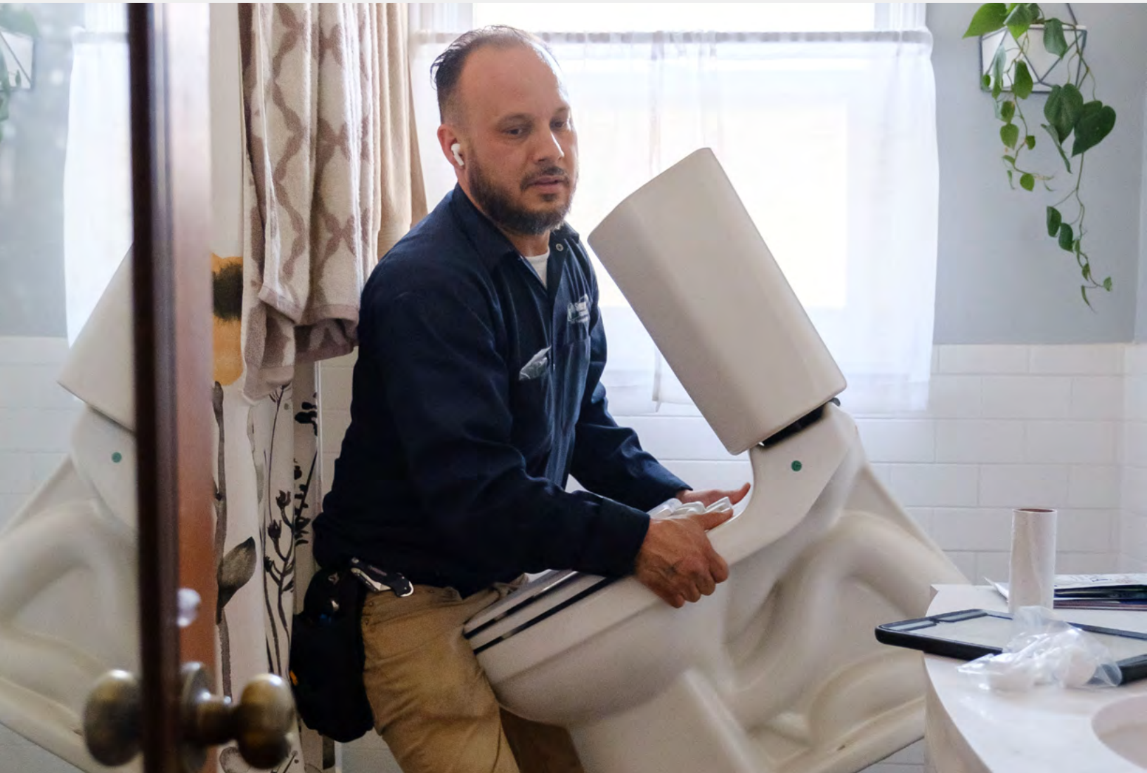
A collaboration with SoCalGas brings waterwise toilets to disadvantaged communities along with irrigation controllers and high-efficiency showerheads.
