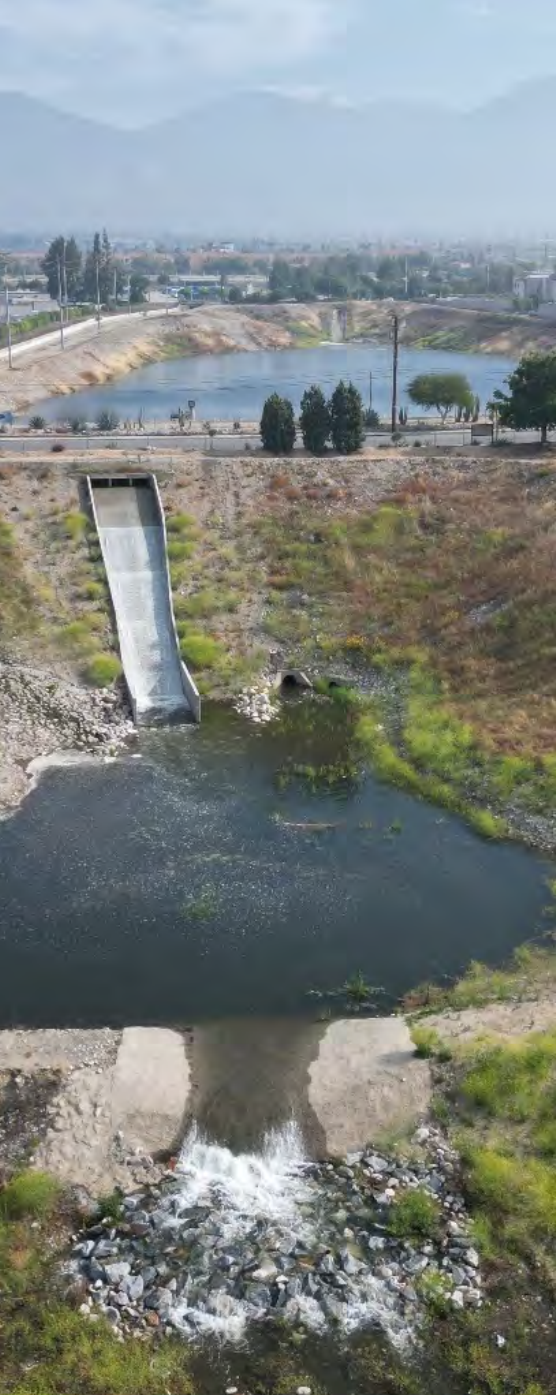
Montclair Basins Improvement Project.
