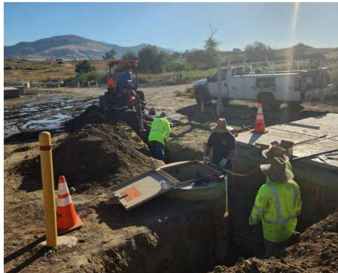
**Staff installing a new piping system to discharge sump water from nearby structures at the Skinner plant**
