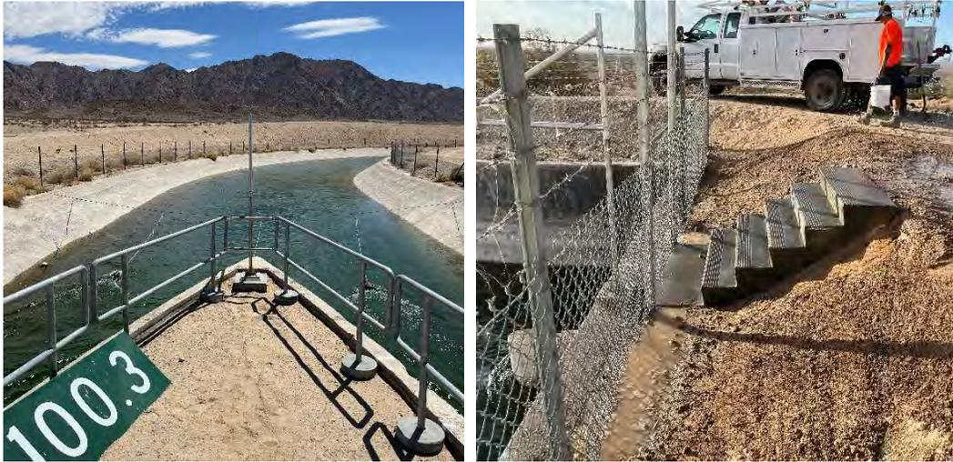
**New transducer bracket and guard rails (left) and new stairs to access a transducer bracket (right) along the CRA**
