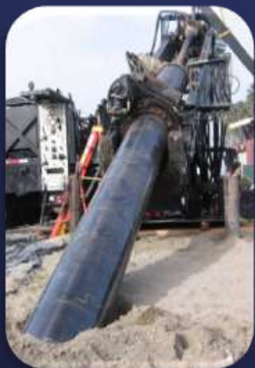
Slant Well Construction
