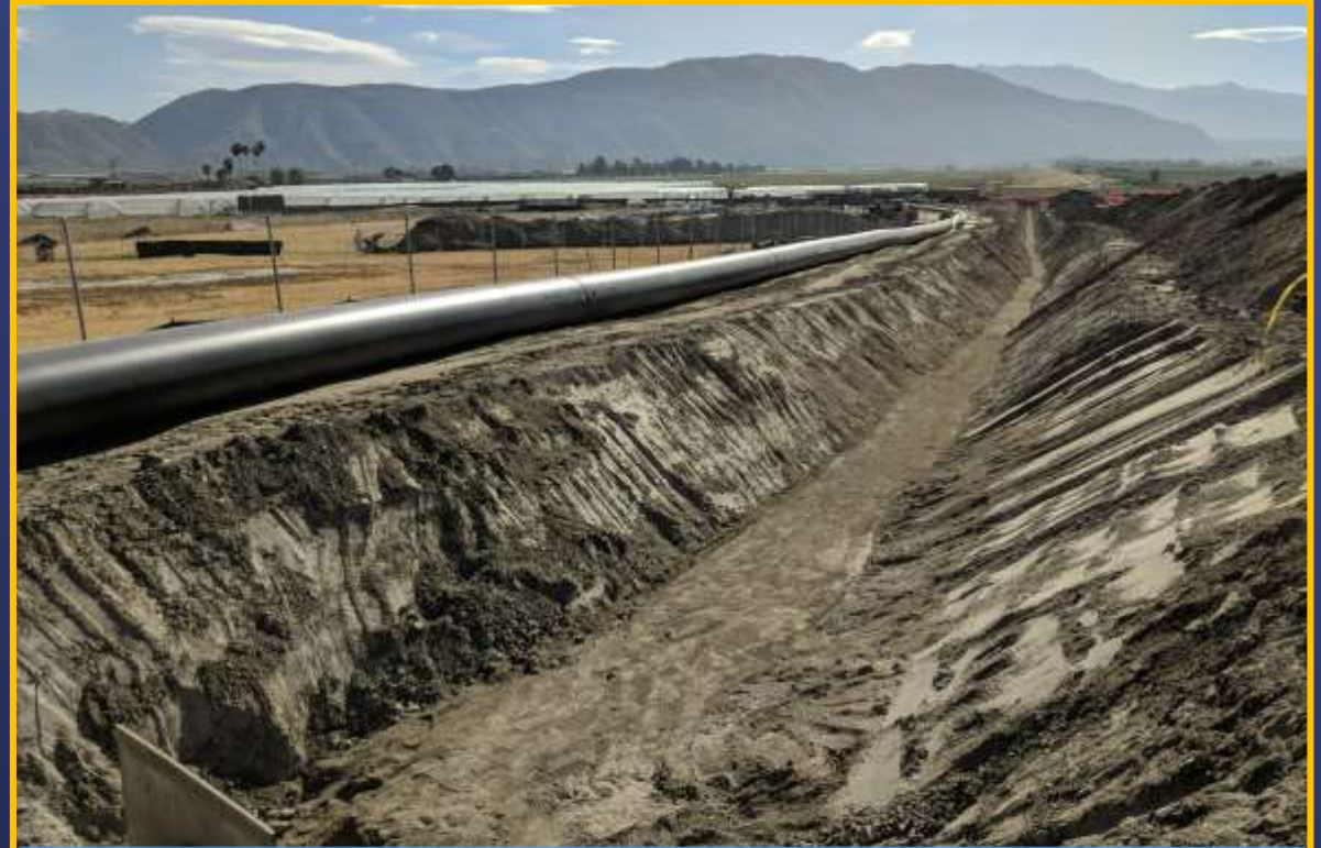
30-inch HDPE Drainage Pipe and Excavation
