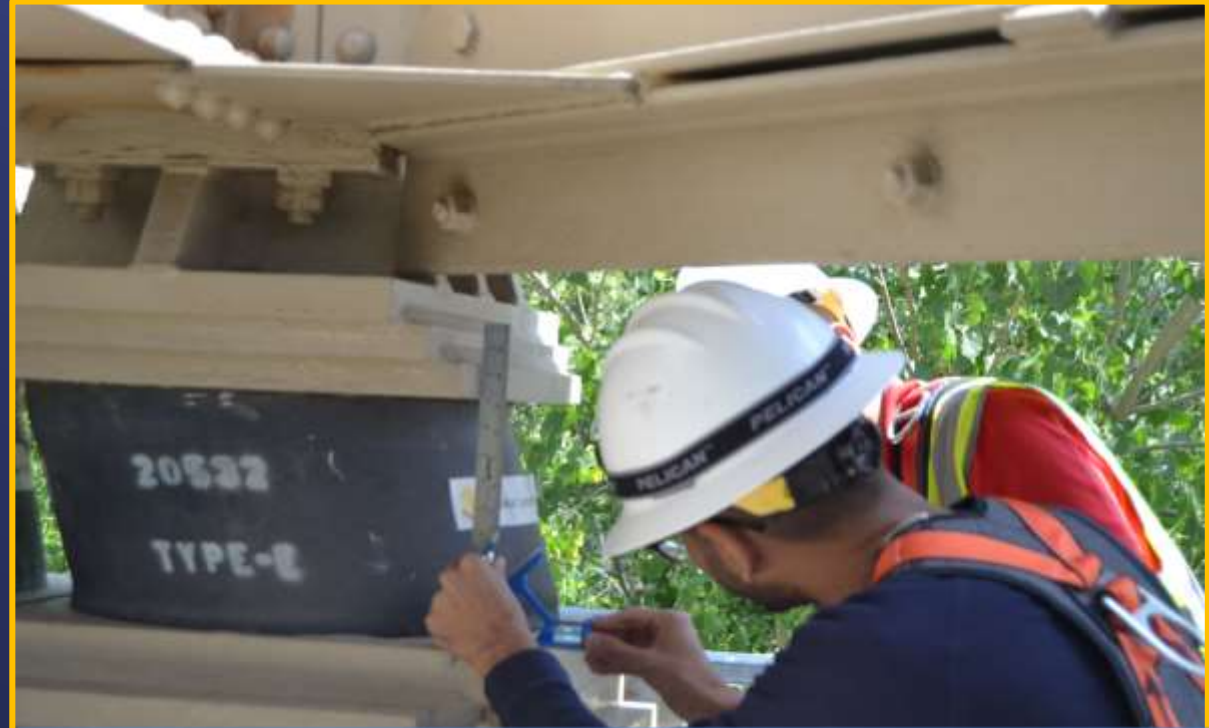
Bridge Base Isolator Inspection
