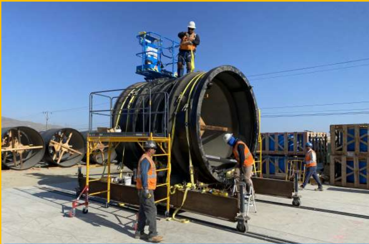
Field Assembly of Kubota ERDIP Sections
