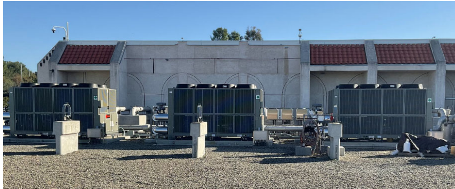
Service Connection OC -88 Chillers Replacement — New Chillers
