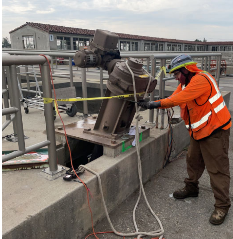
Weymouth Basins 5–8 and Filter Building No. 2 Rehabilitation — Beginning Demolition of the Filter Drain Valves, North of Filter Building No. 2
