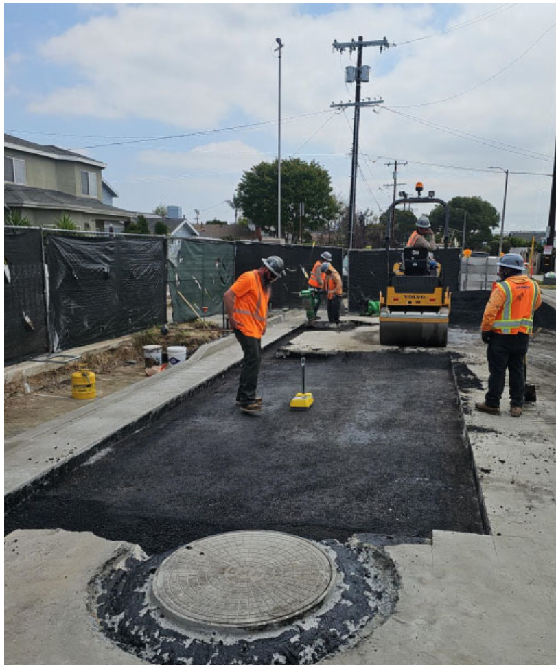
Second Lower Feeder PCCP Rehabilitation Reach 3B Metropolitan Staff Asphalt Compaction Testing
