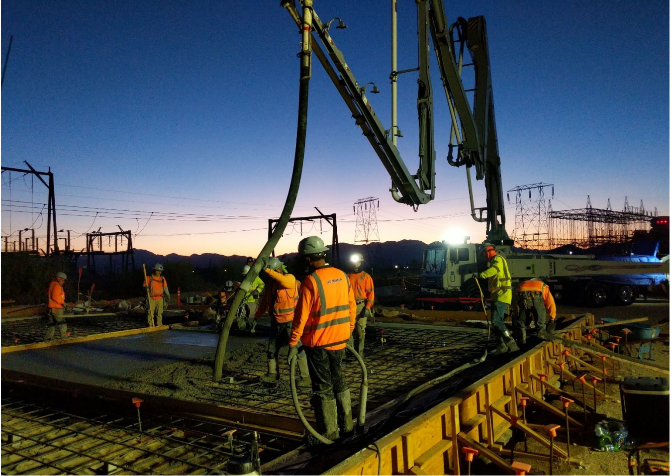
CRA Storage Buildings—Placing Concrete for Storage Building Slab at Eagle Mountain Pump Plant
