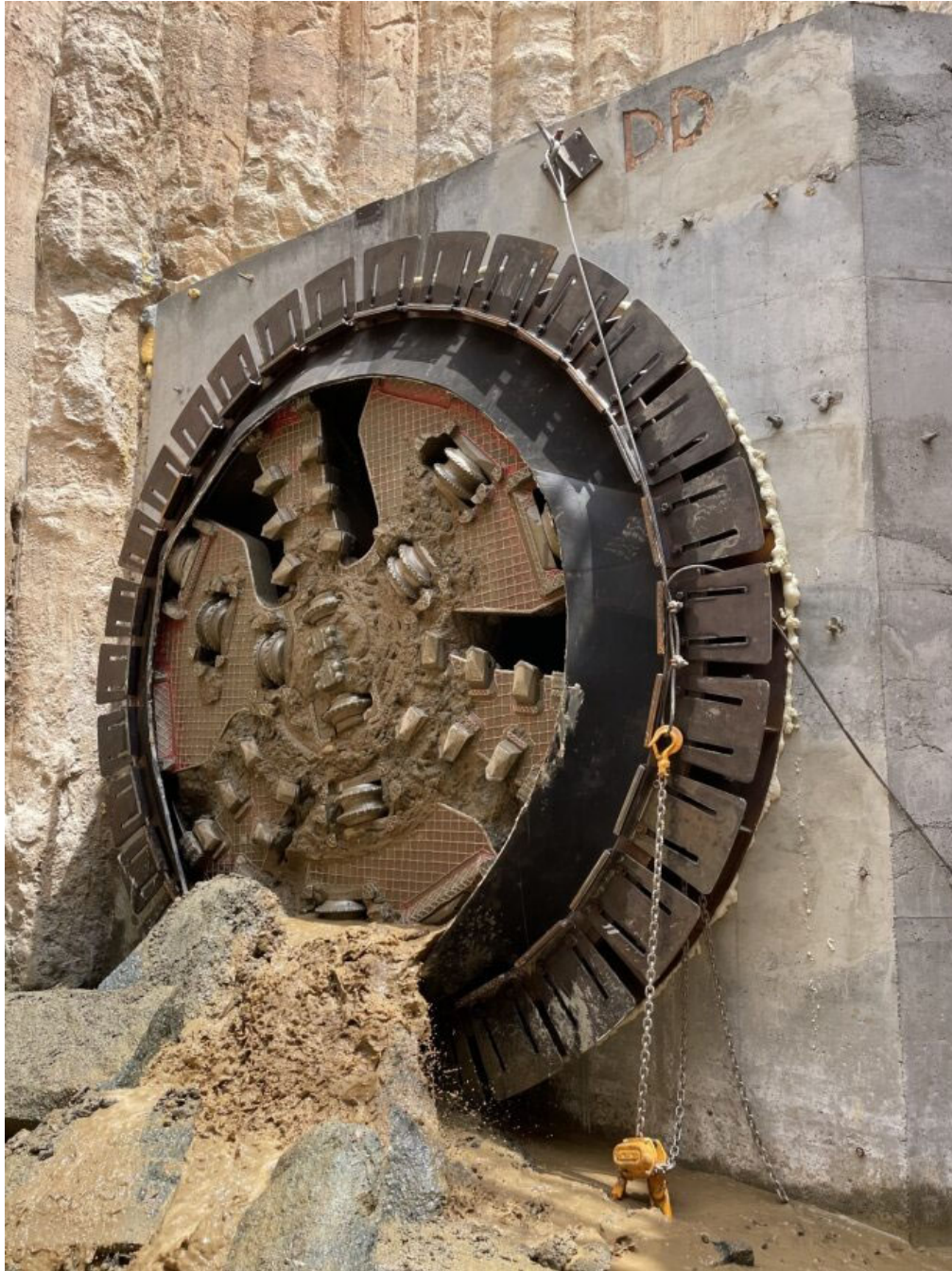
Perris Valley Pipeline—Hole-through TBM at second shaft
