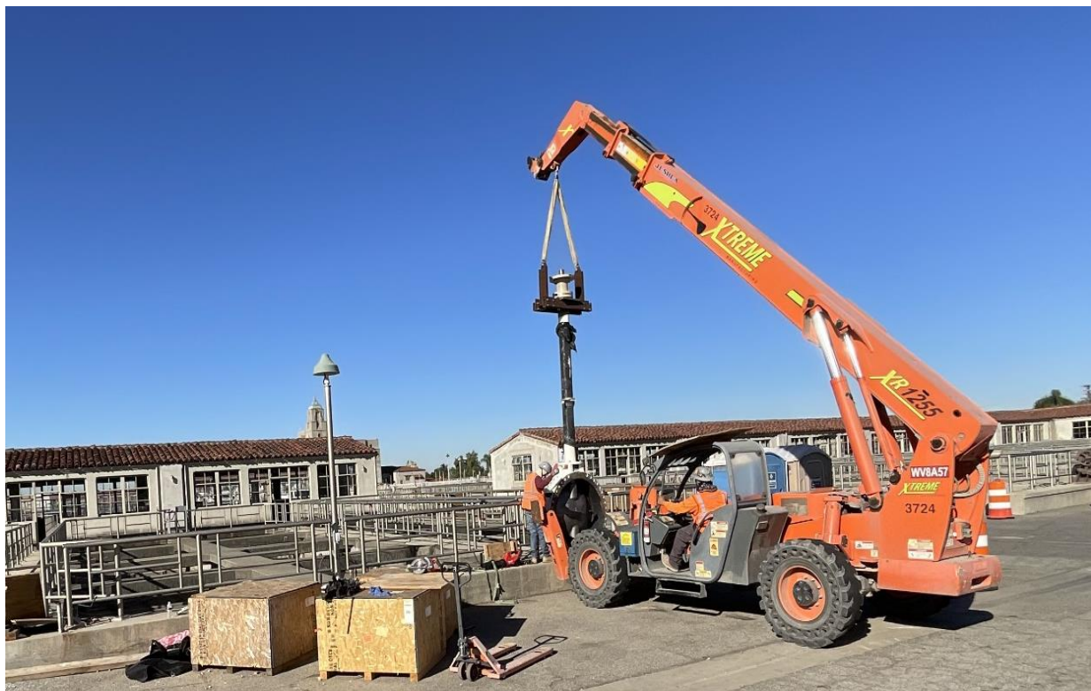
Installing a new drain valve on the north side of Filter Building No. 2
