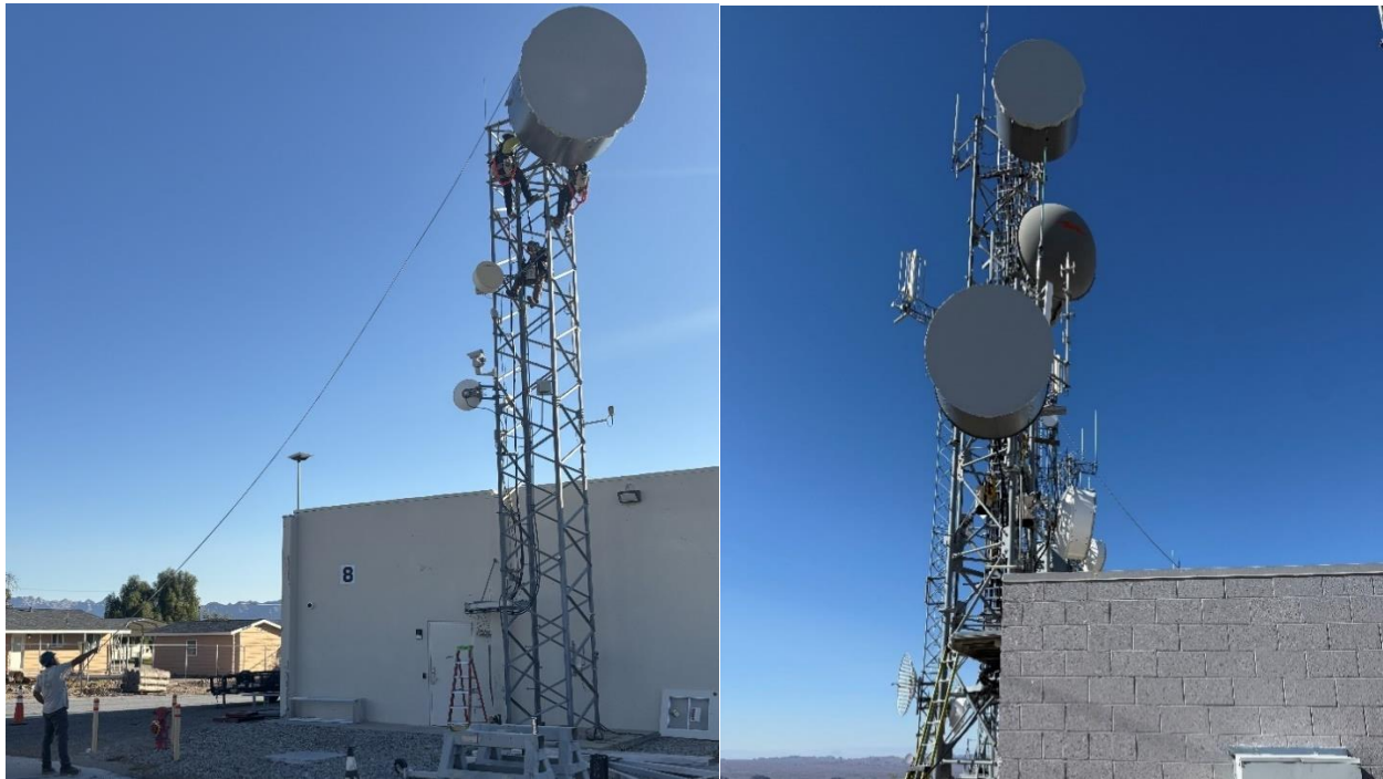
Installation of microwave antenna and waveguide on existing communication tower at Eagle Mountain Pumping Plant (left) and Chuckwalla site (right)
