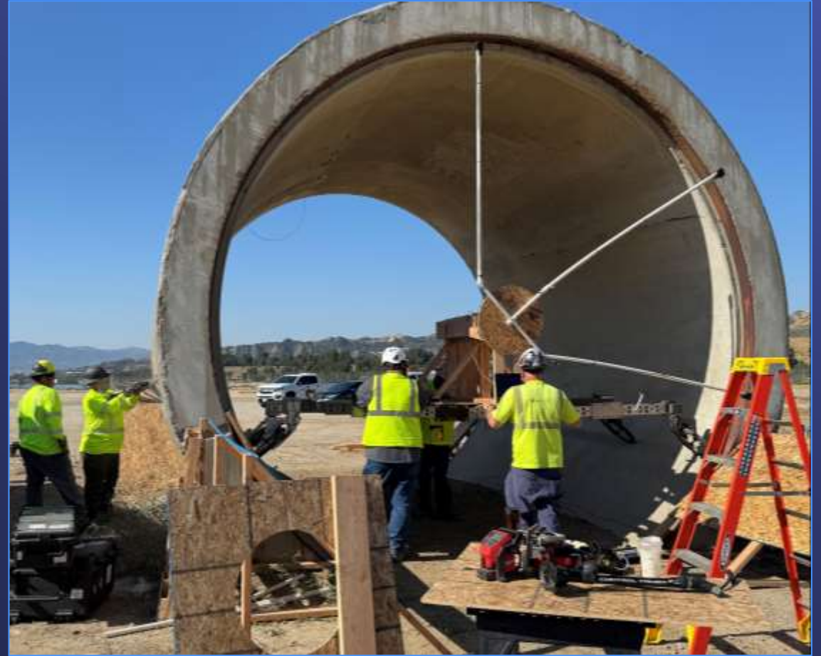
Calibration of PipeDiver® Tool For 201-inch Diameter Pipe at Foothill PCS
