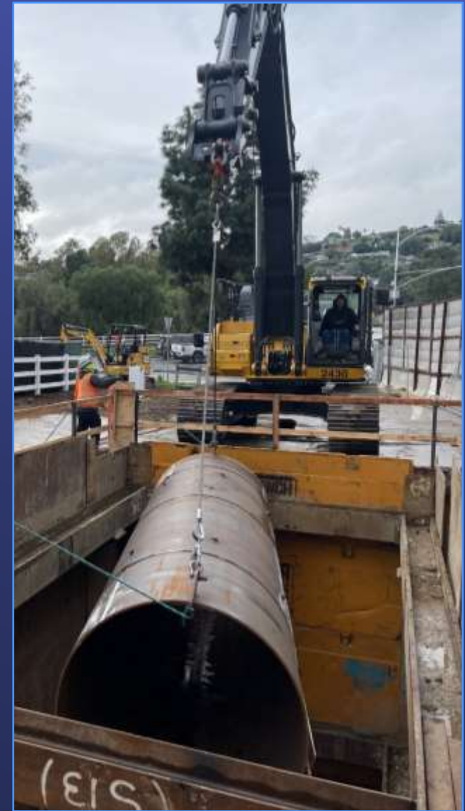
Second Lower Feeder Relining
