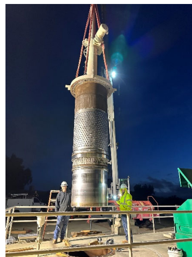
Staff removing a 42-inch sleeve valve at Auld Valley Control Structure on San Diego Pipeline No. 3
