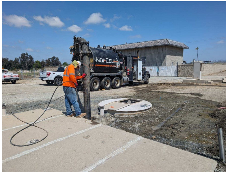
Contractor assisting with vacuum excavation at the EM-17 service connection
