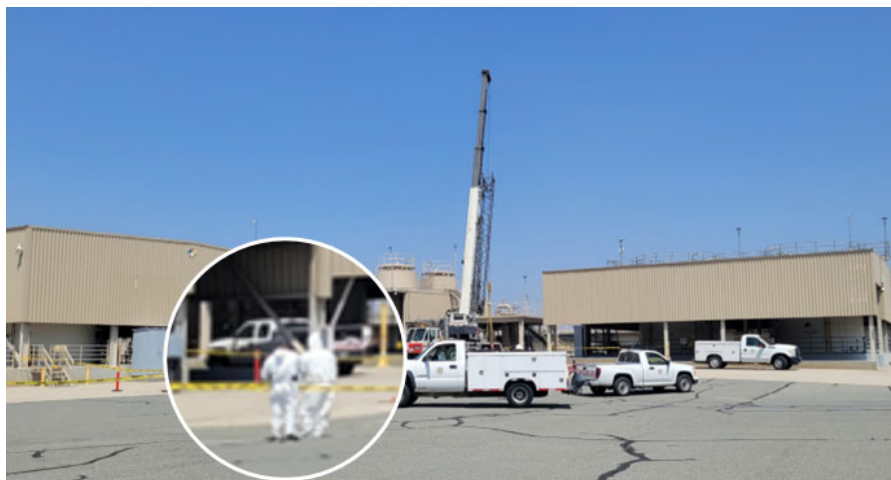
Staff in personal protective equipment investigating the exact location of the ammonia leak at the Mills plant
