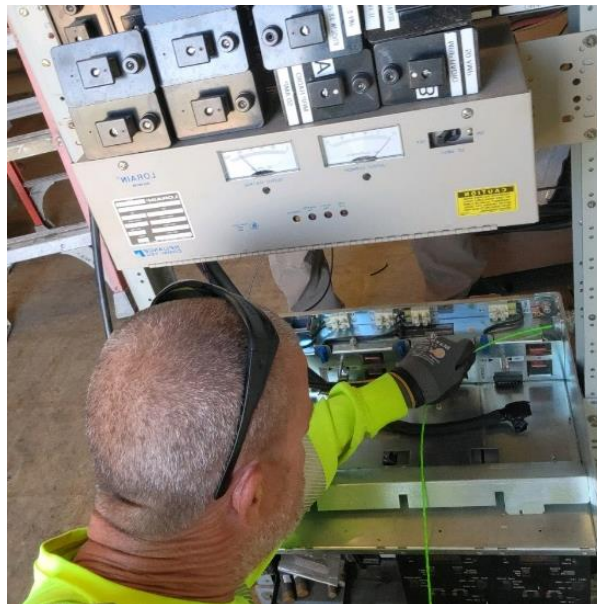
Staff installing the new rectifier system at the Detention Peak communications site
