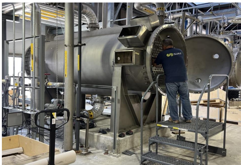
Contractor installing new dielectrics for the ozone generators at the Jensen plant
