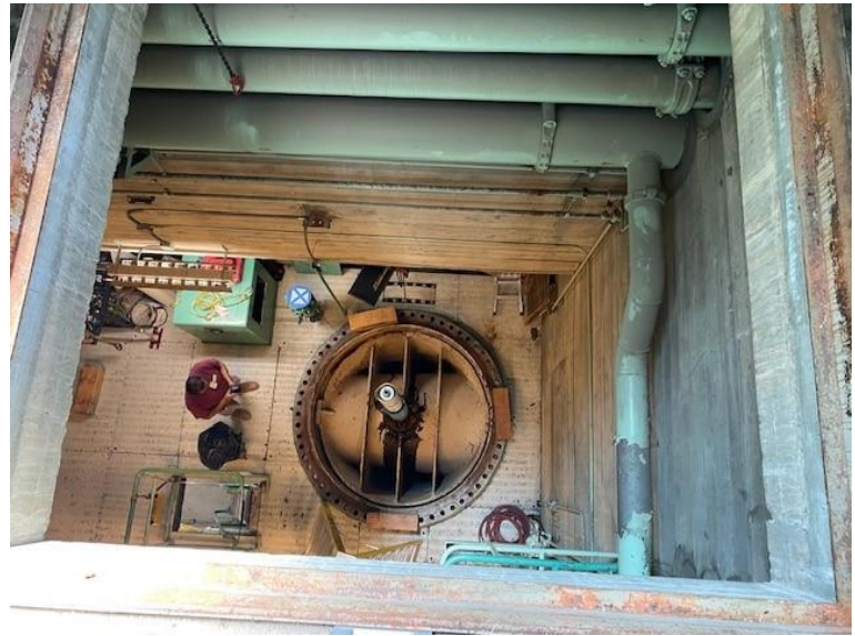
Discharge Valve repair at Gene pumping plant
