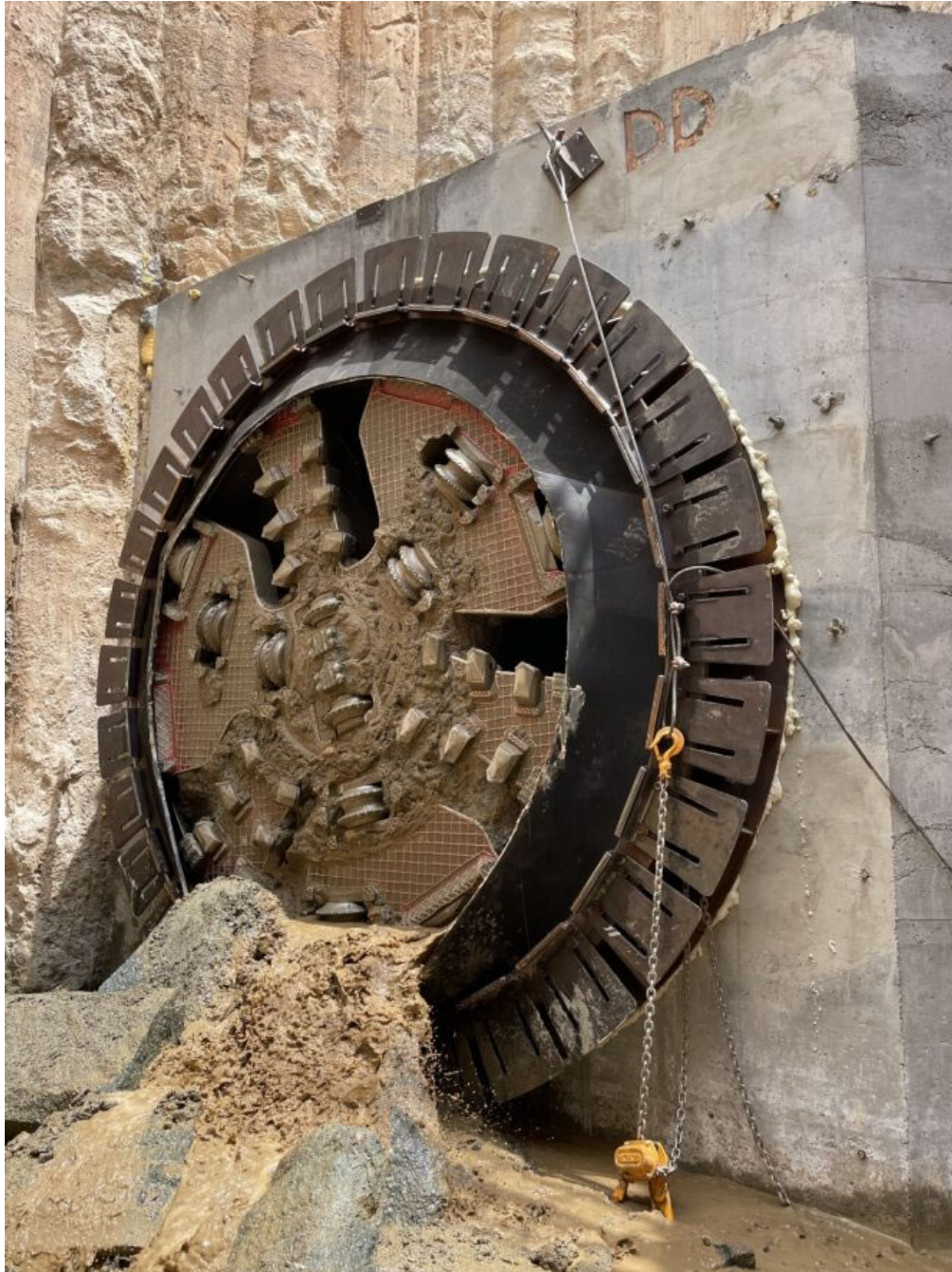
Perris Valley Pipeline—Hole-through TBM at second shaft
