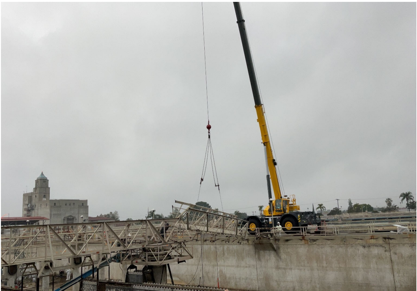
Weymouth Basins 5-8 and Filter Building No. 2 Rehabilitation—Weymouth Basin 5 Bridge Demolition
