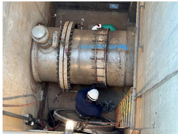
Staff installing orifice plate at USG-03 service connection
