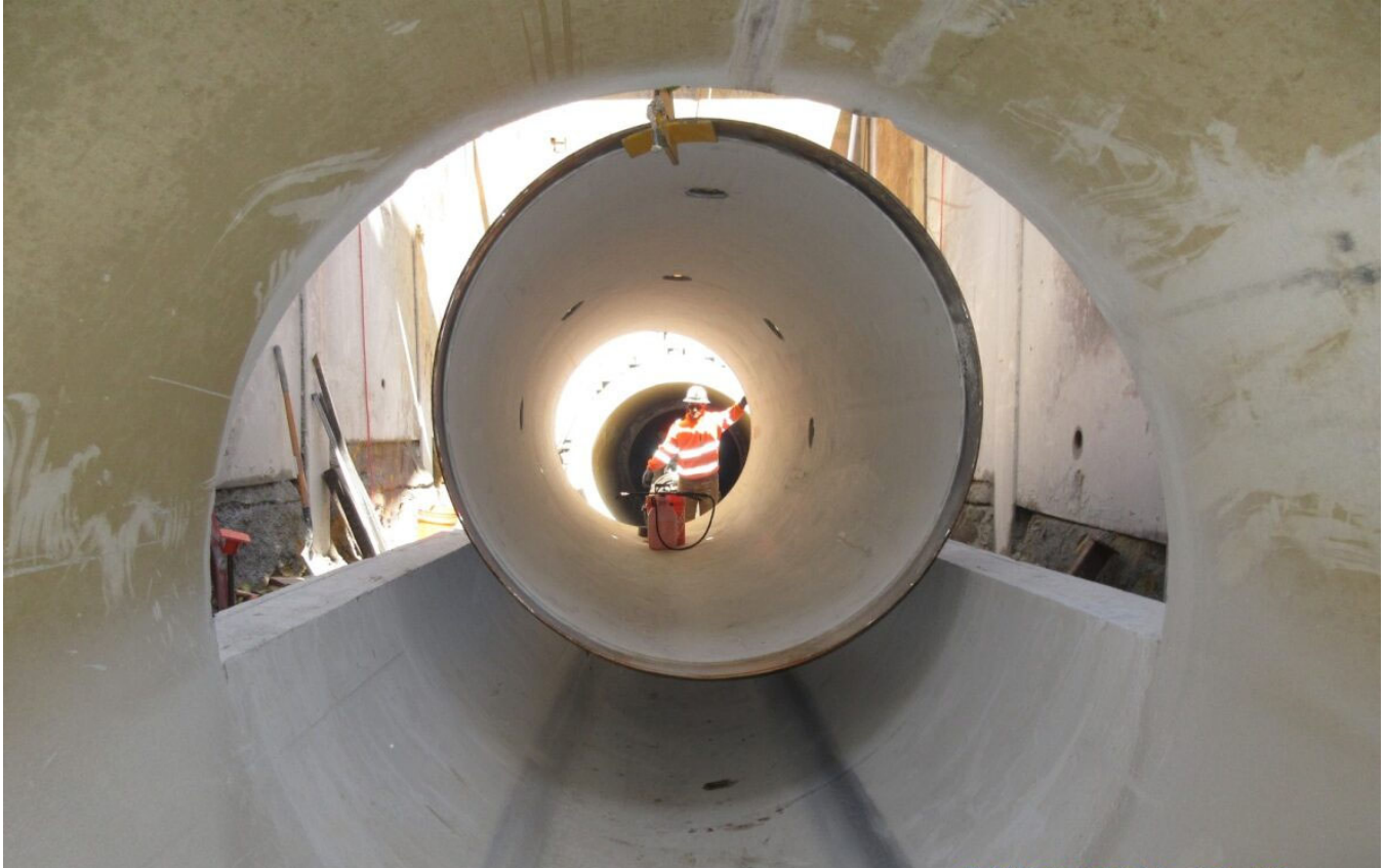
Allen-McColloch Pipeline Urgent Relining—New pipe liner installation
