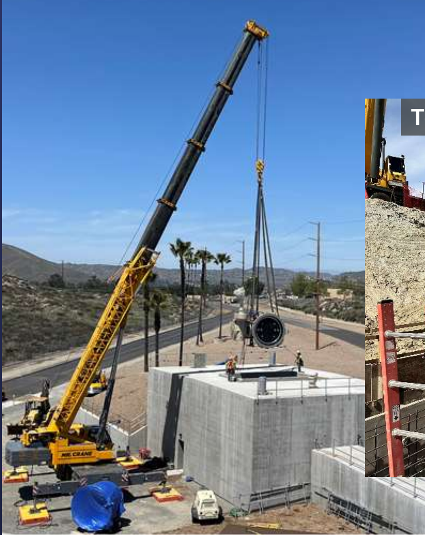
Valve Installation at Wadsworth Bypass
