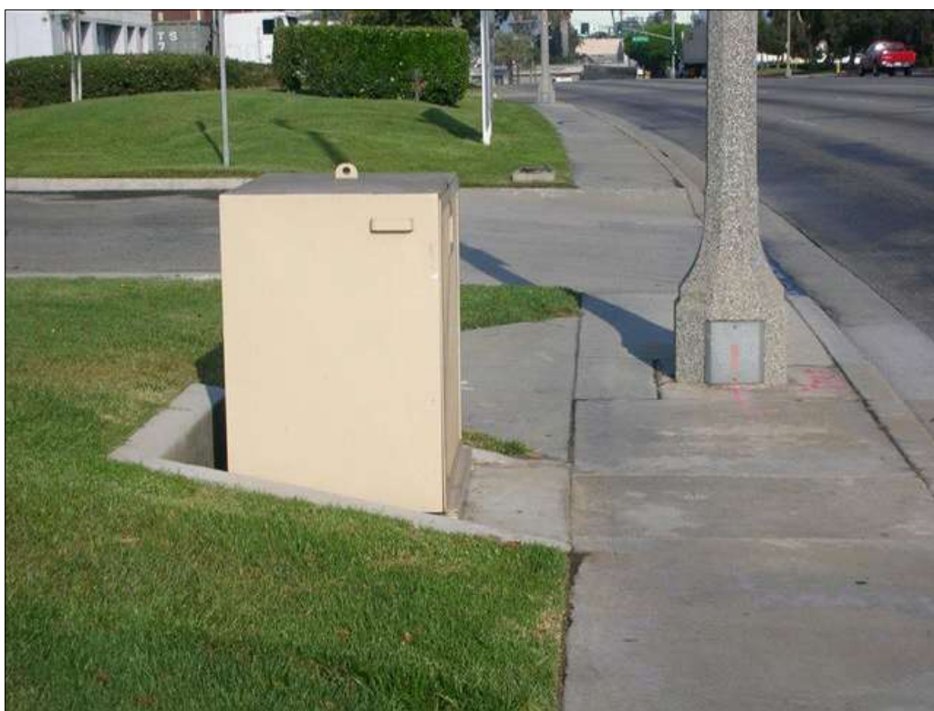
Figure 5. Typical Above Ground ARVV Enclosure
