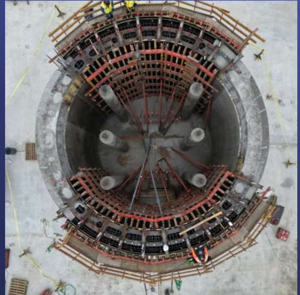
Surge Tank Foundation
