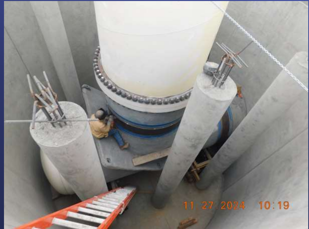
Surge Tank Foundation Pipe Installation
