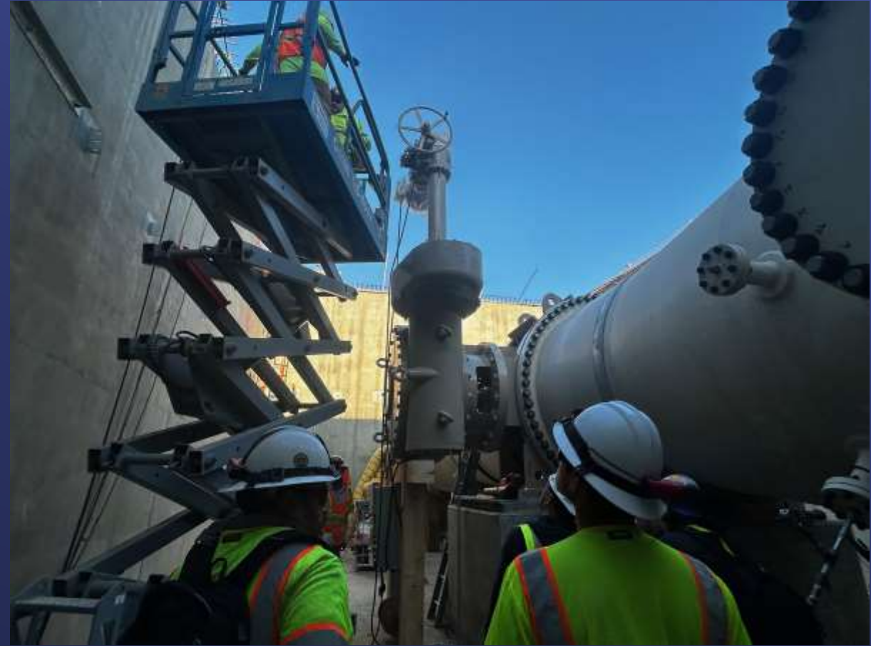
84-Inch Diameter Valve Fit Up
