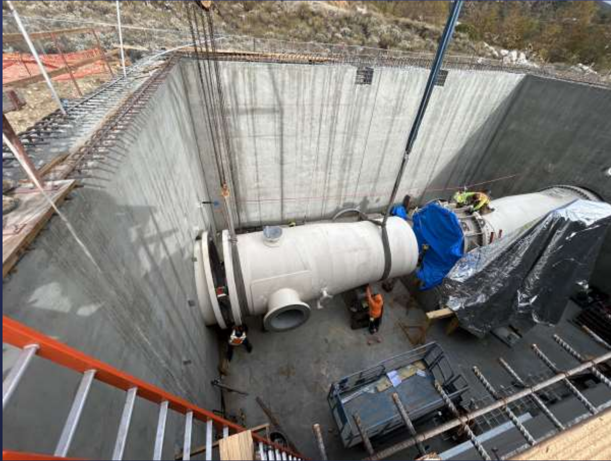
Pipe Reducer Installation
