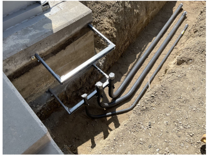
Staff installing electrical conduits for the heli-hydrant at the Diemer plant.
