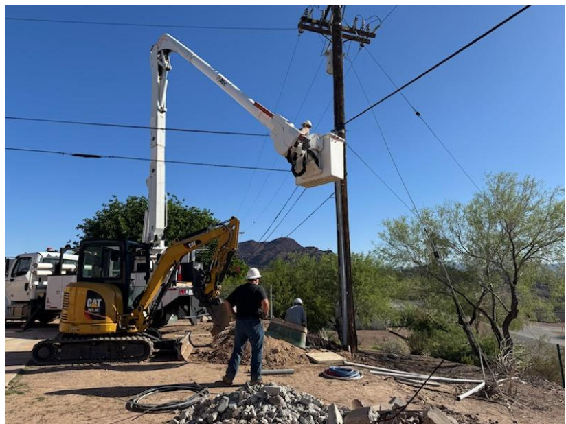
Staff installing a new electrical service line at Gene.
