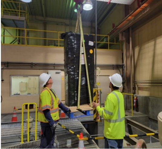
Staff moving new UPS unit into position (left) and making electrical connections (right) at San Dimas PCS.
