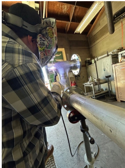
Staff welding new piping (left) and new piping and fixtures (right) for the Iron Mountain domestic water tank.
