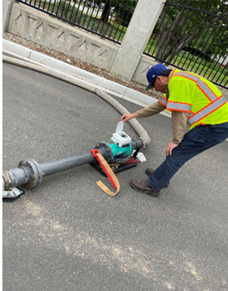
Staff verifying flow rate for the air gap to the sanitary sewer at the Weymouth plant.
