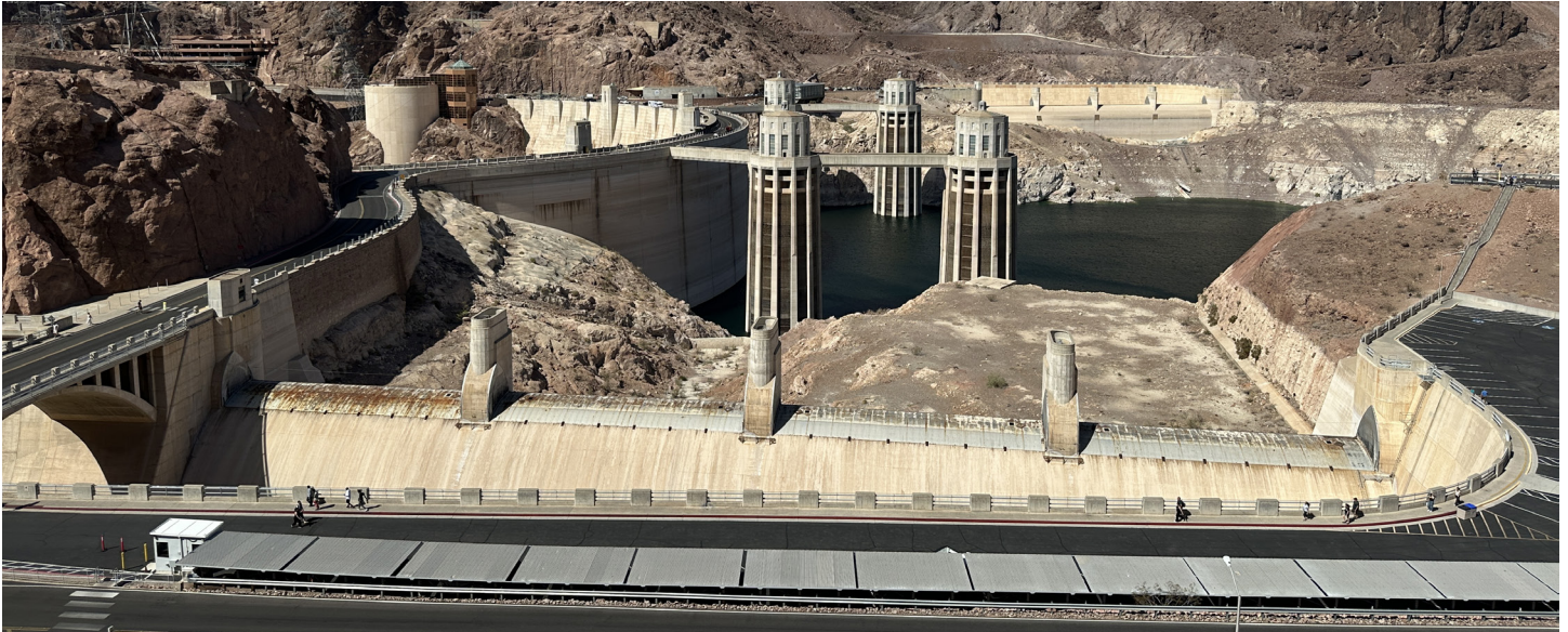
Hoover Dam Arizona spillway, photo by Connie Castle, Department of Interior.
