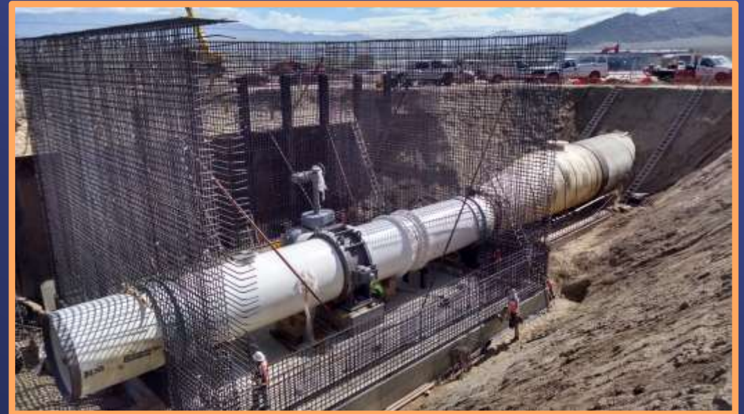
IF to Lakeview Vault Construction
