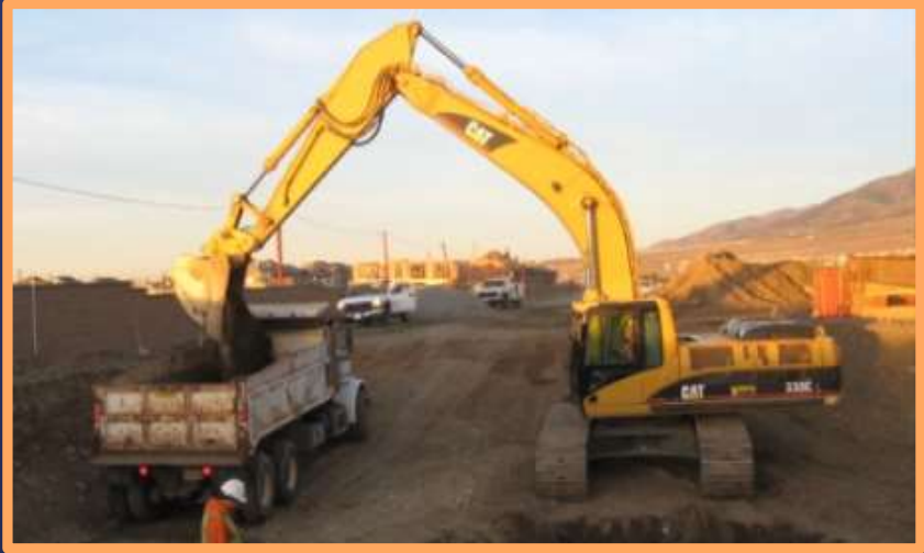
Tracking Heavy Equipment for Immediate Mobilization
