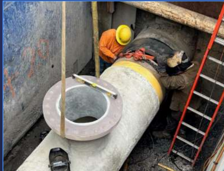
Installing Closure Piece
