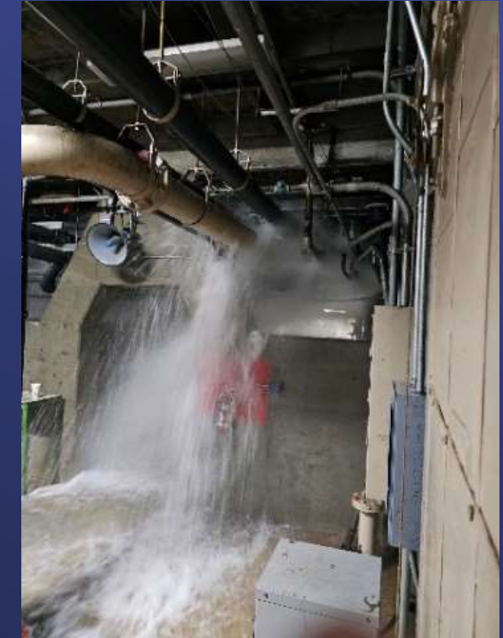
Weymouth Domestic Water Line Leak June 2024
