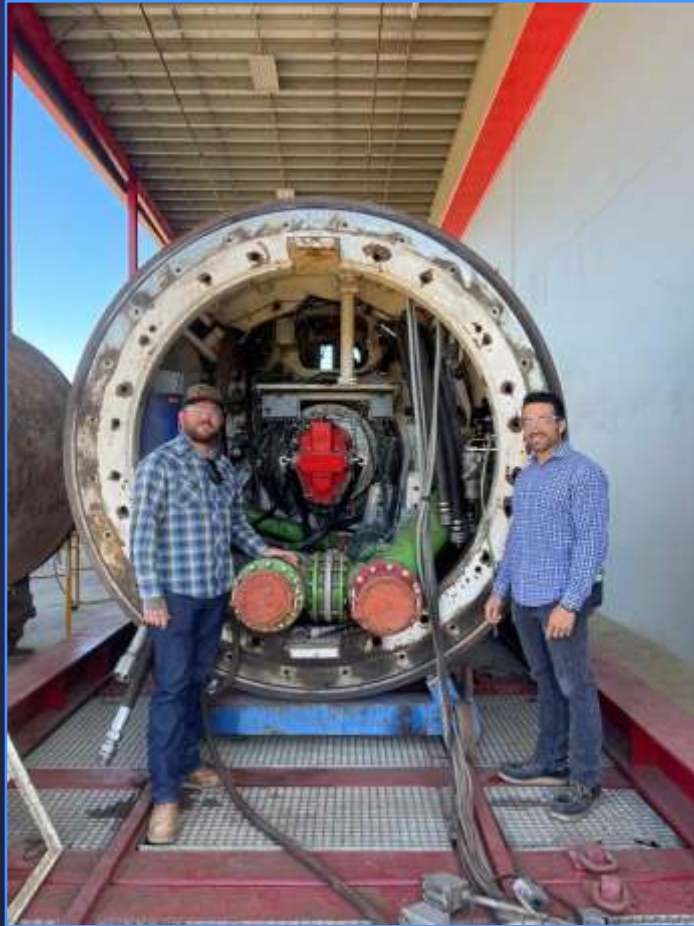
Staff inspection of TBM refurbishment
