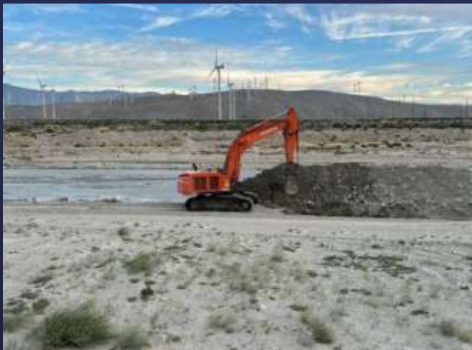
Repairing Whitewater Conveyance Channel
