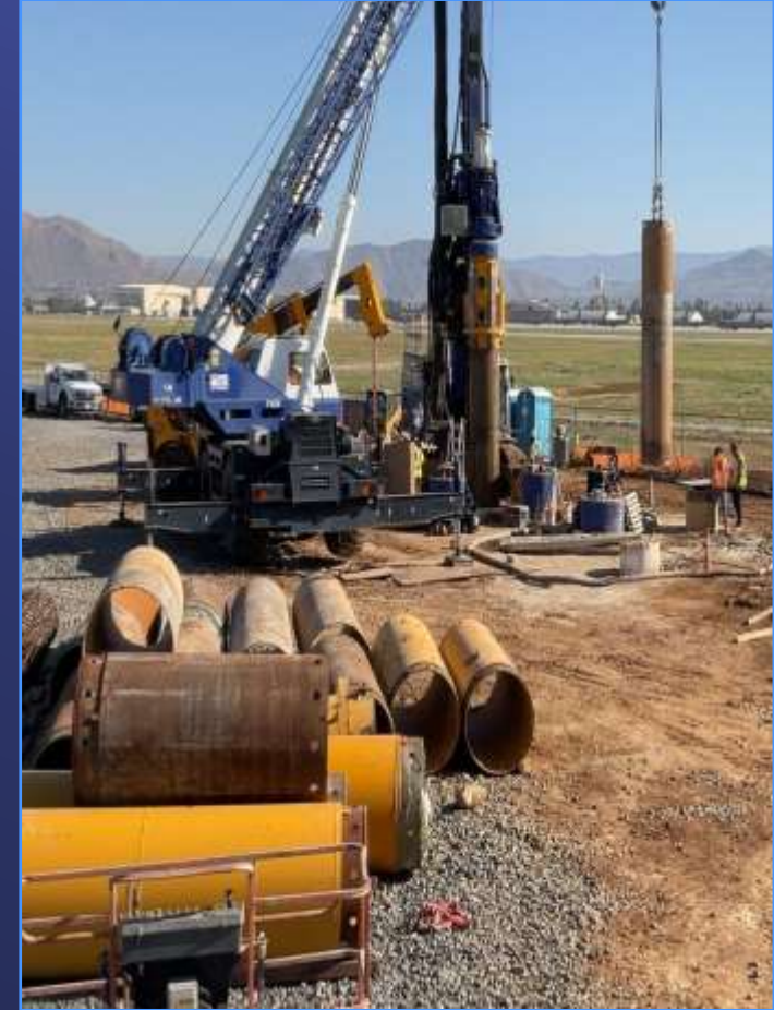
Contractor drilling shaft piles
