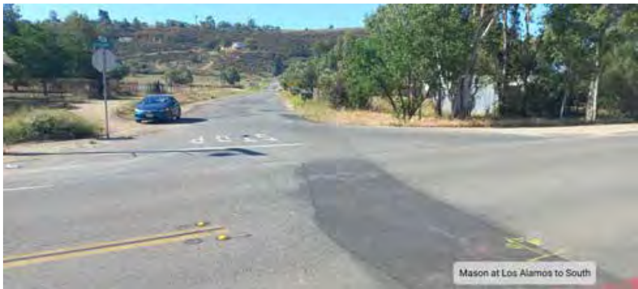
Photograph No. 11: Mason Avenue at Los Alamos Road, facing south.
