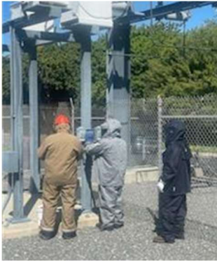
Staff performing High voltage switching practical operations (left) and reporting the completion of switching (right) at Coyote Creek HEP.
