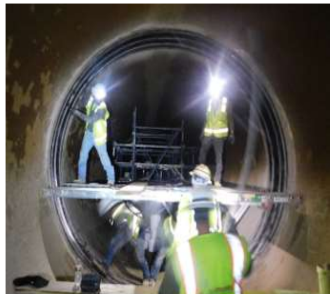
Freda Siphon Weko Seal Installation
