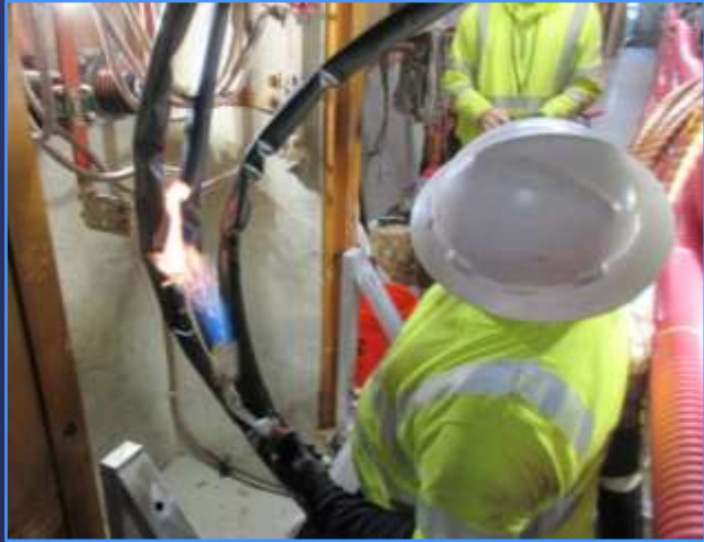
Application of heat to the termination kit
