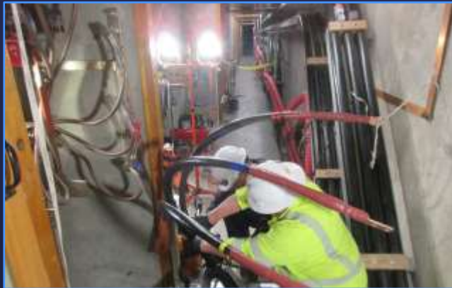
Switch house cable installation
