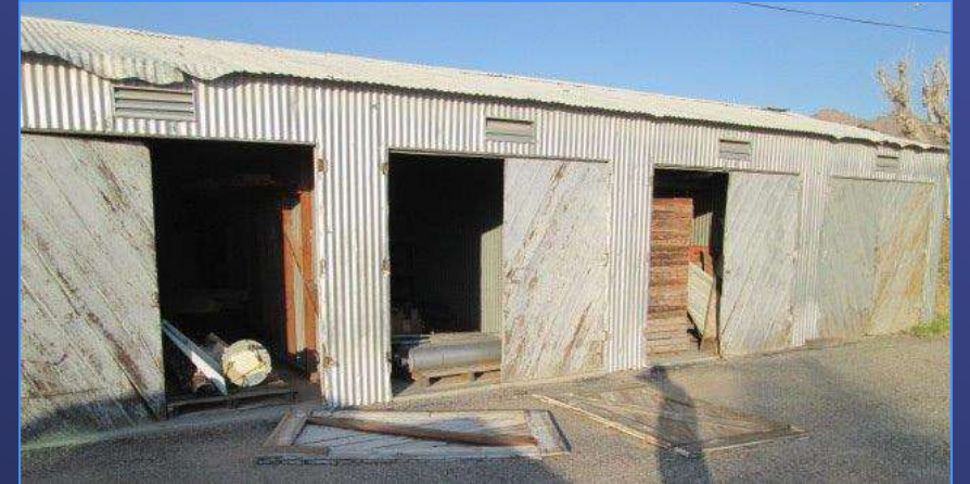
Iron Mtn. Storage Building (Existing)
