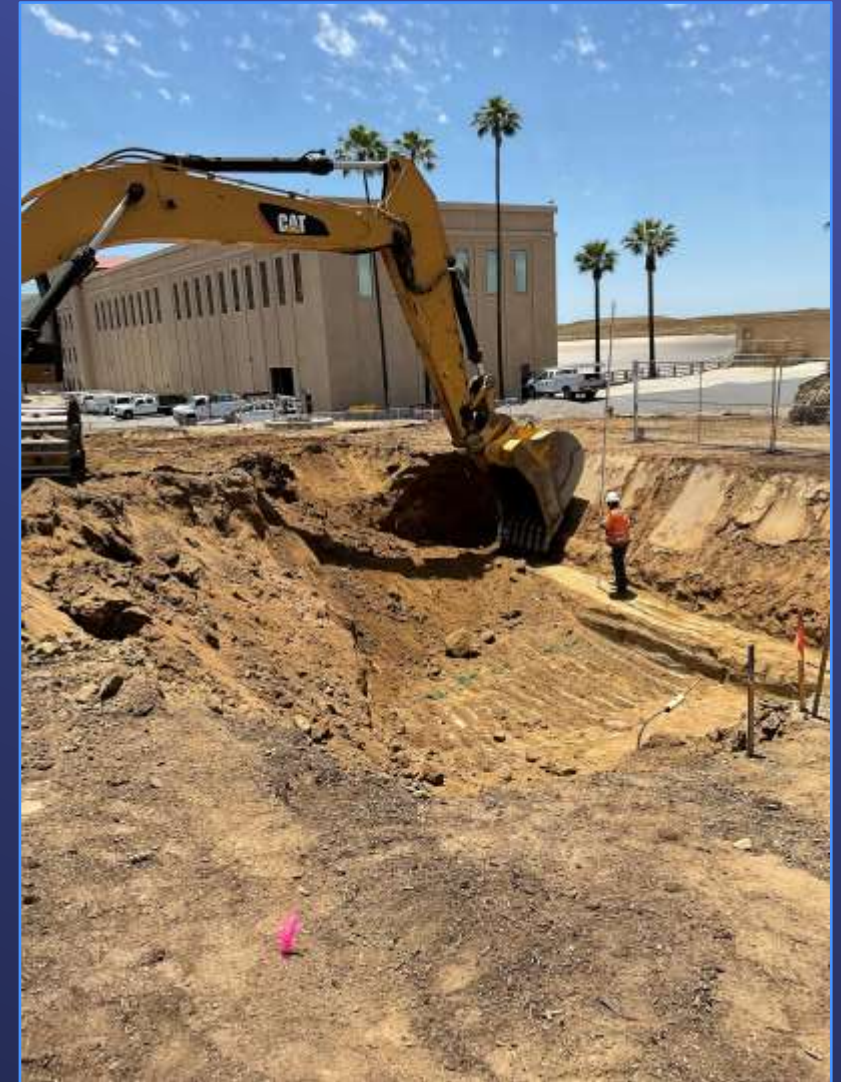
Wadsworth Pumping Plant Intertie: Excavation for valve structure
