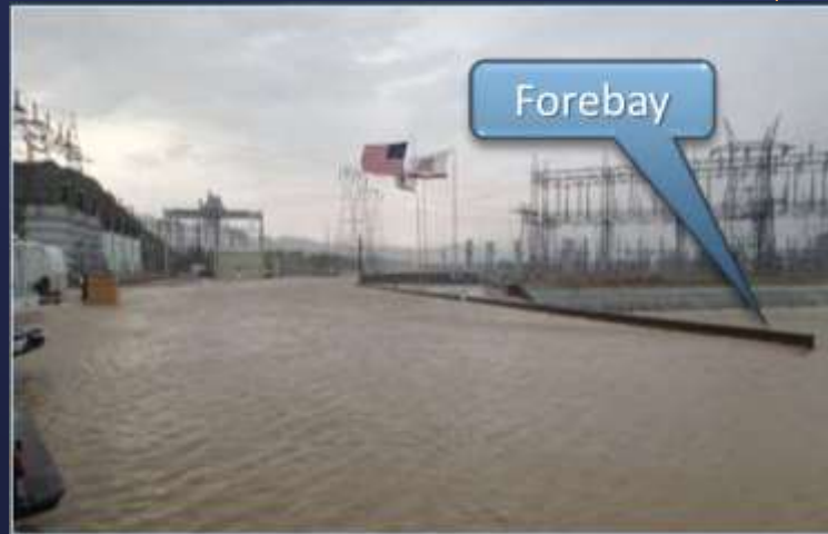
Eagle Mtn. Pumping Plant Storm Inundation
