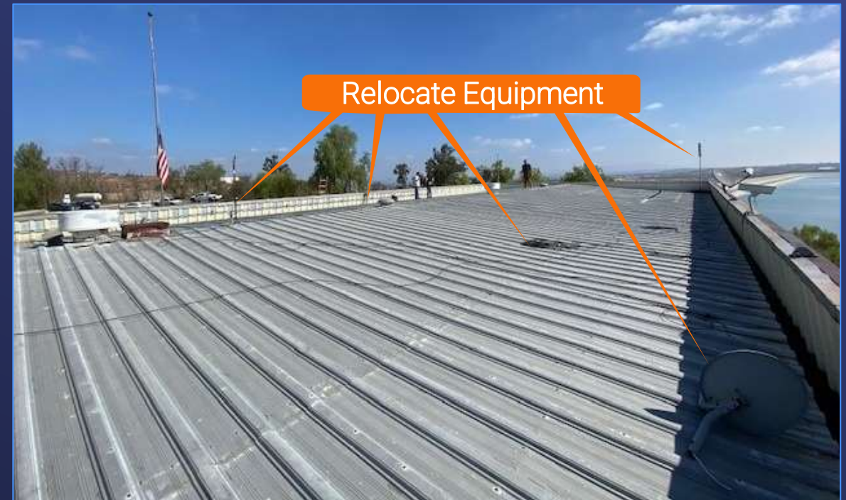
Metropolitan Force Construction
