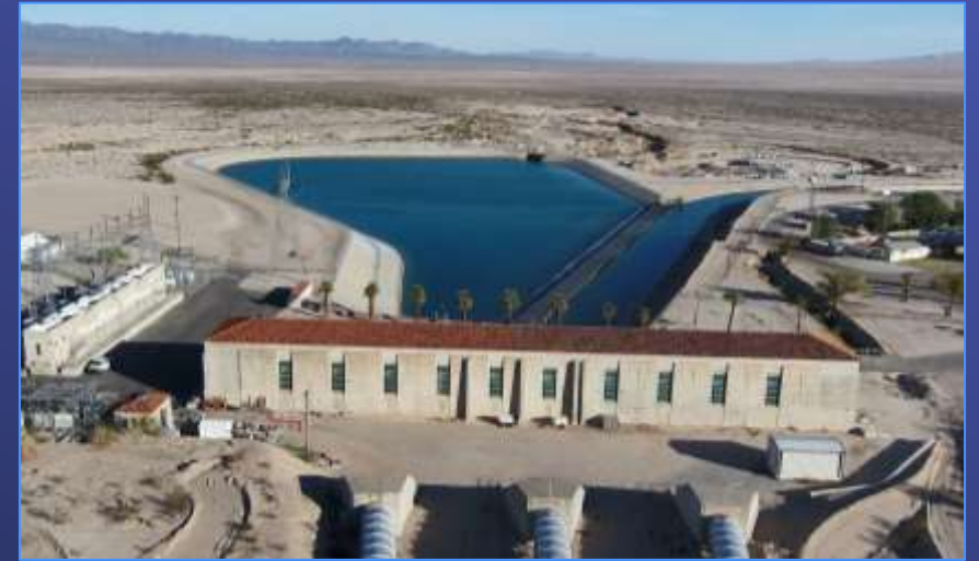
Iron Mountain Pumping Plant
