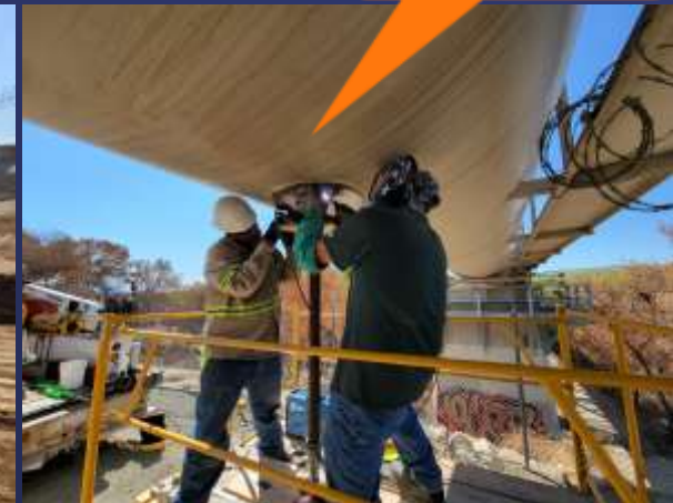
6-inch Valve Installation
