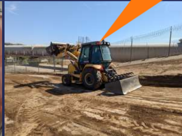
Clearing and Grading for Crane Pad
