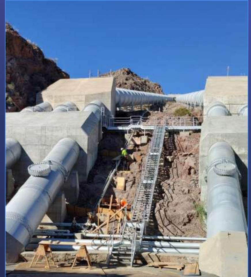
Contractor prepared subgrade to install above-ground conduit support pedestals at Intake Pumping Plant
