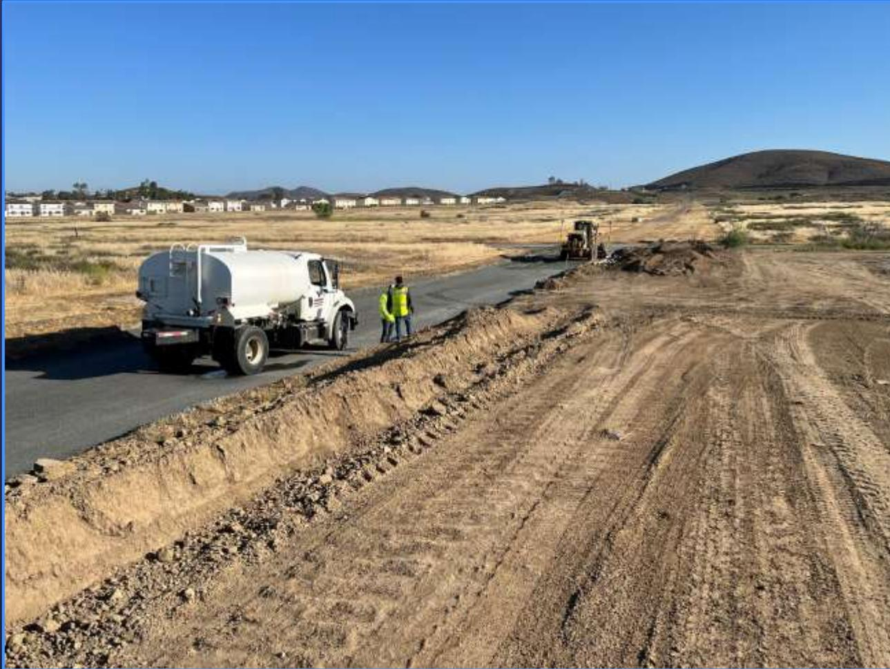
Contractor installing crushed aggregate base for fire access road at Skinner WTP
