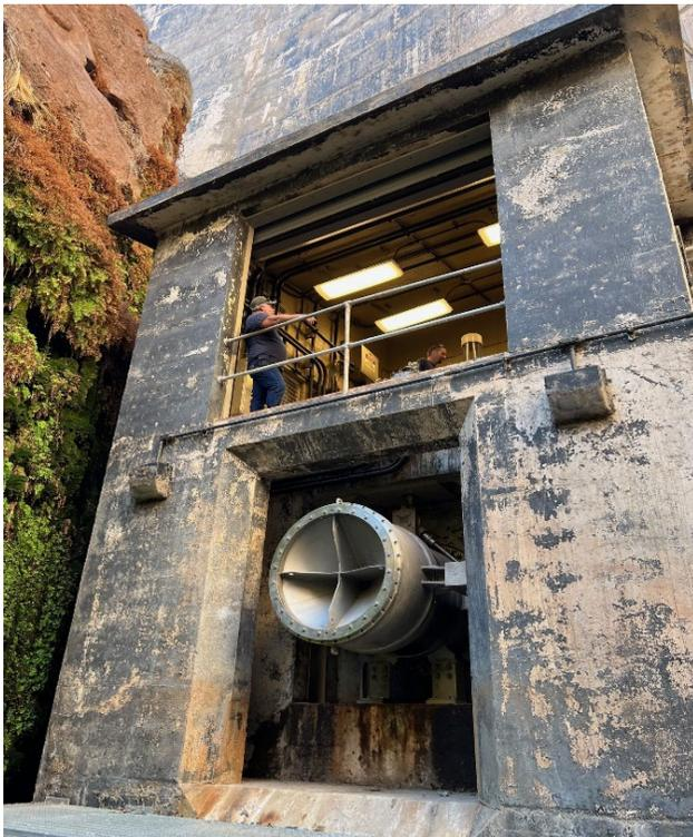
*Fig 1: Photo of conical valve sitting inside the Valve House*
