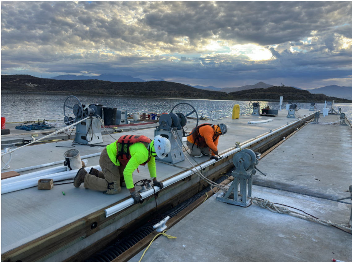
Diamond Valley Lake (DVL) Wave Attenuator Replacement — Installation of Vinyl Rub Strip on New Floating Wave Attenuator
