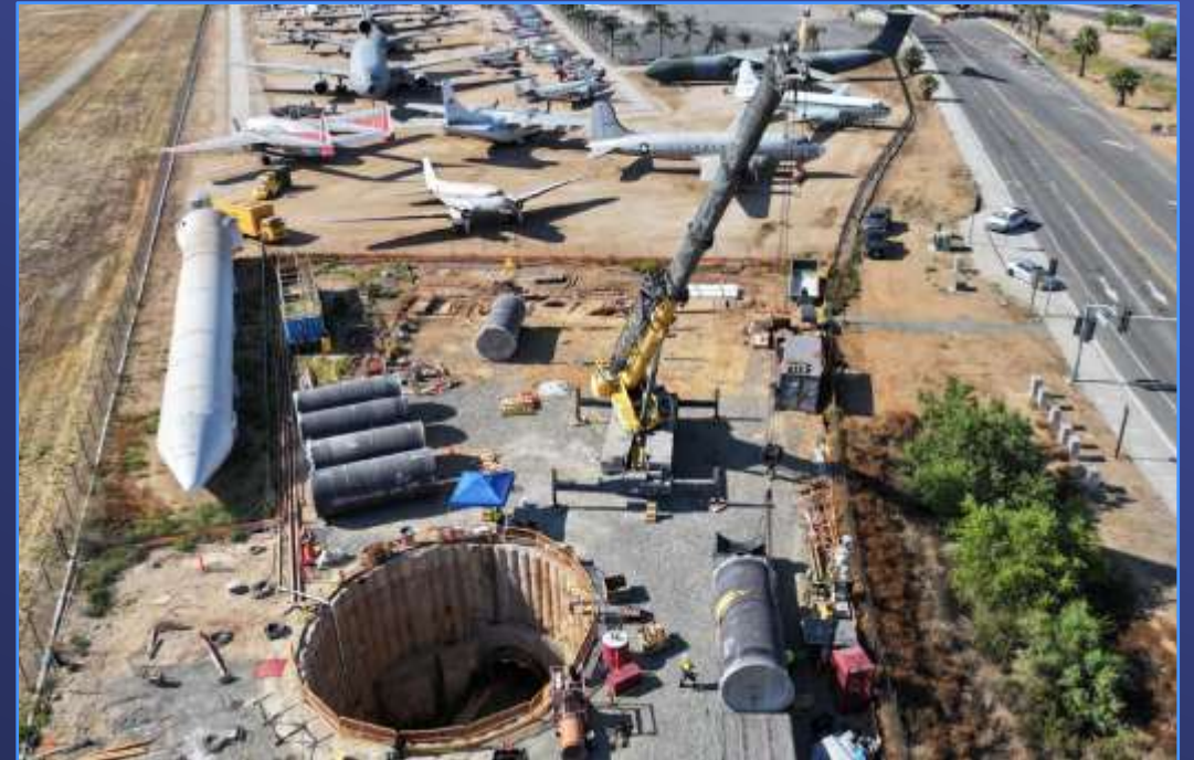
Perris Valley Pipeline I-215 Crossing
