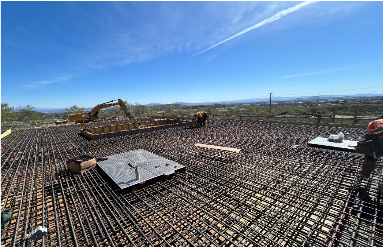
Installation of reinforcing steel at a valve vault structure deck at the DWR Devil Canyon facility
