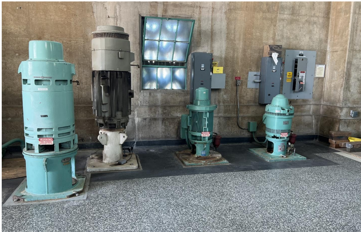
Circulating water and sump pumps at Hinds Pumping Plant
