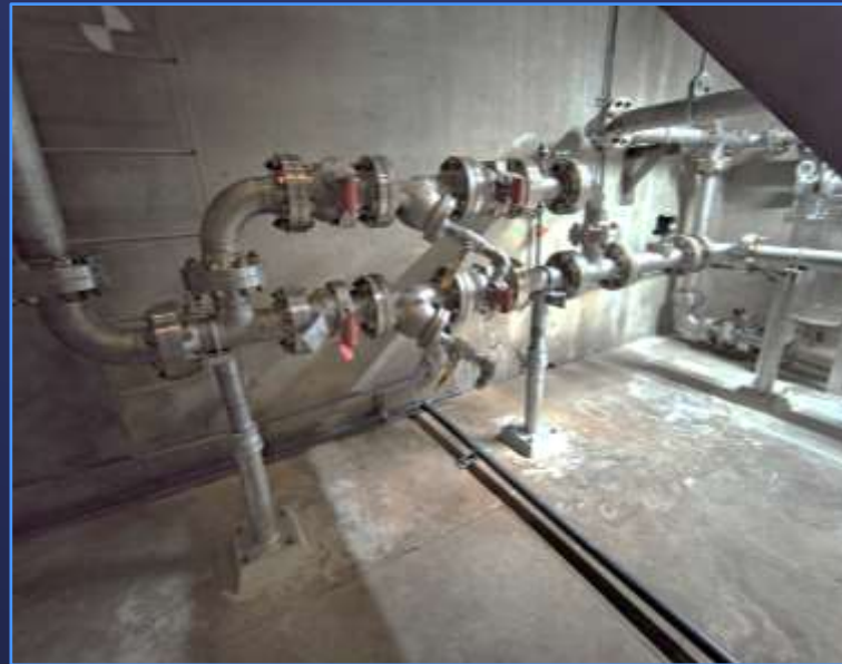
Red Mountain HEP Cooling Water System Rehabilitation
