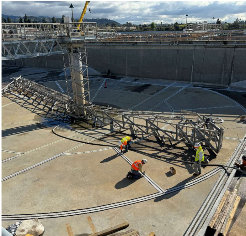
Weymouth Basins 5–8 and Filter Building No. 2 Rehabilitation—Installing Joint Sealant at Basin 7
