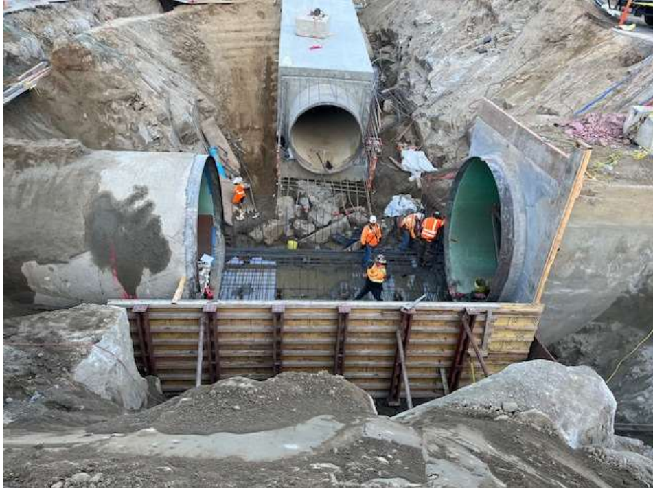
Wadsworth Pumping Plant Bypass— Constructing Forms For Encasement at the Tee Section
