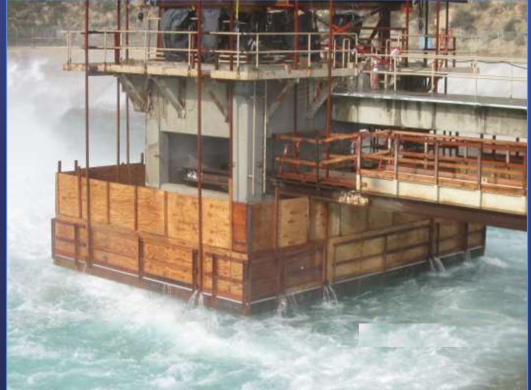
Working on Outlet Tower while Forebay in Service
