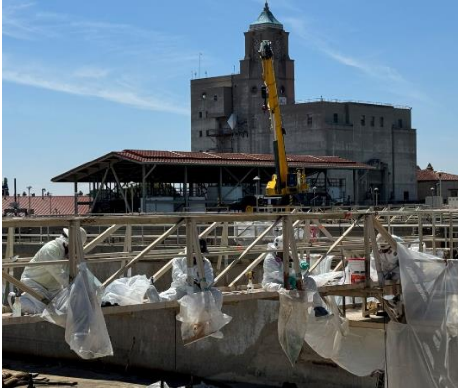
Weymouth Basins 5–8 and Filter Building No. 2 Rehabilitation Coating abatement at Basin 6 clarifier bridges
