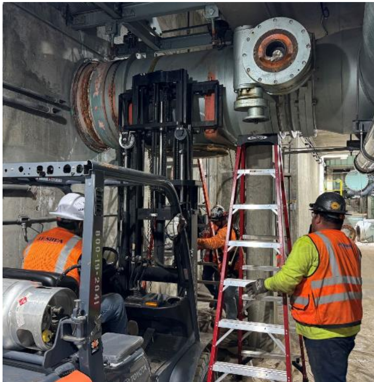
Weymouth Basins 5–8 and Filter Building No. 2 Rehabilitation Dismantling backwash piping at filter gallery for installation of new 30-inch backwash valve
