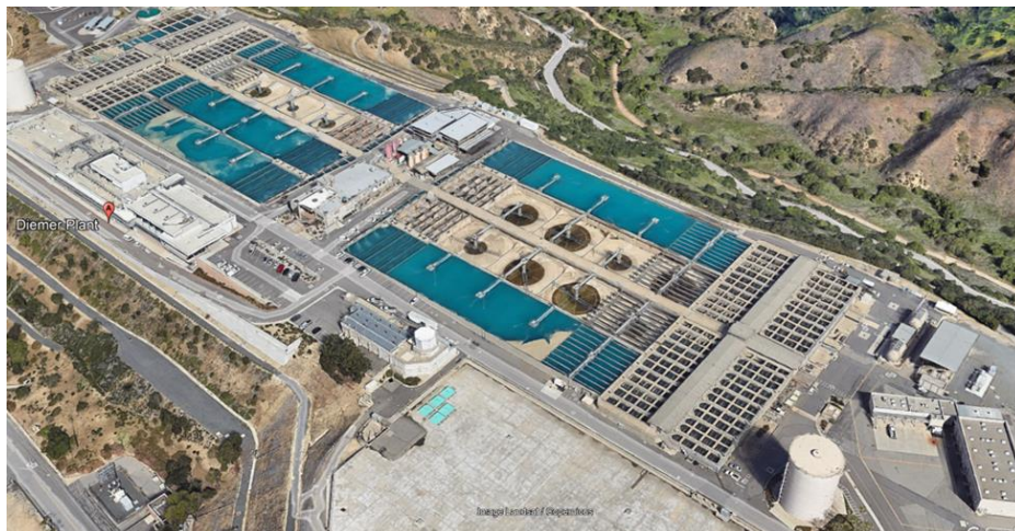
Robert B. Diemer Water Treatment Plant
