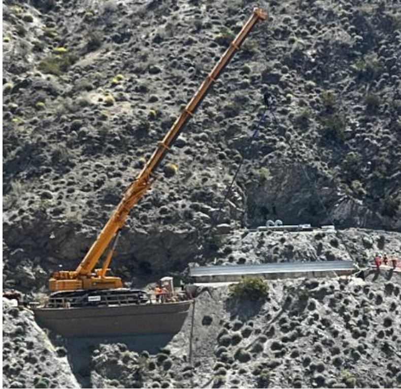
Conduit Structural Protection—Concrete girder installation at aqueduct tunnel portal access road
