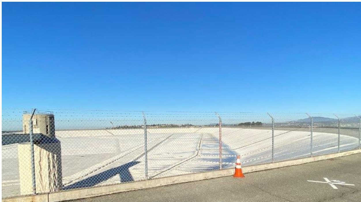
View of the existing Garvey Reservoir floating cover and outlet tower
