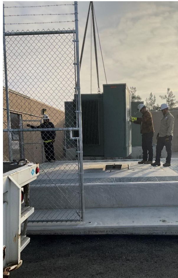
Installation of new HVAC system on the ozone switchgear building rooftop (Left) and transformer on the foundation inside the RPU switchyard (Right)
