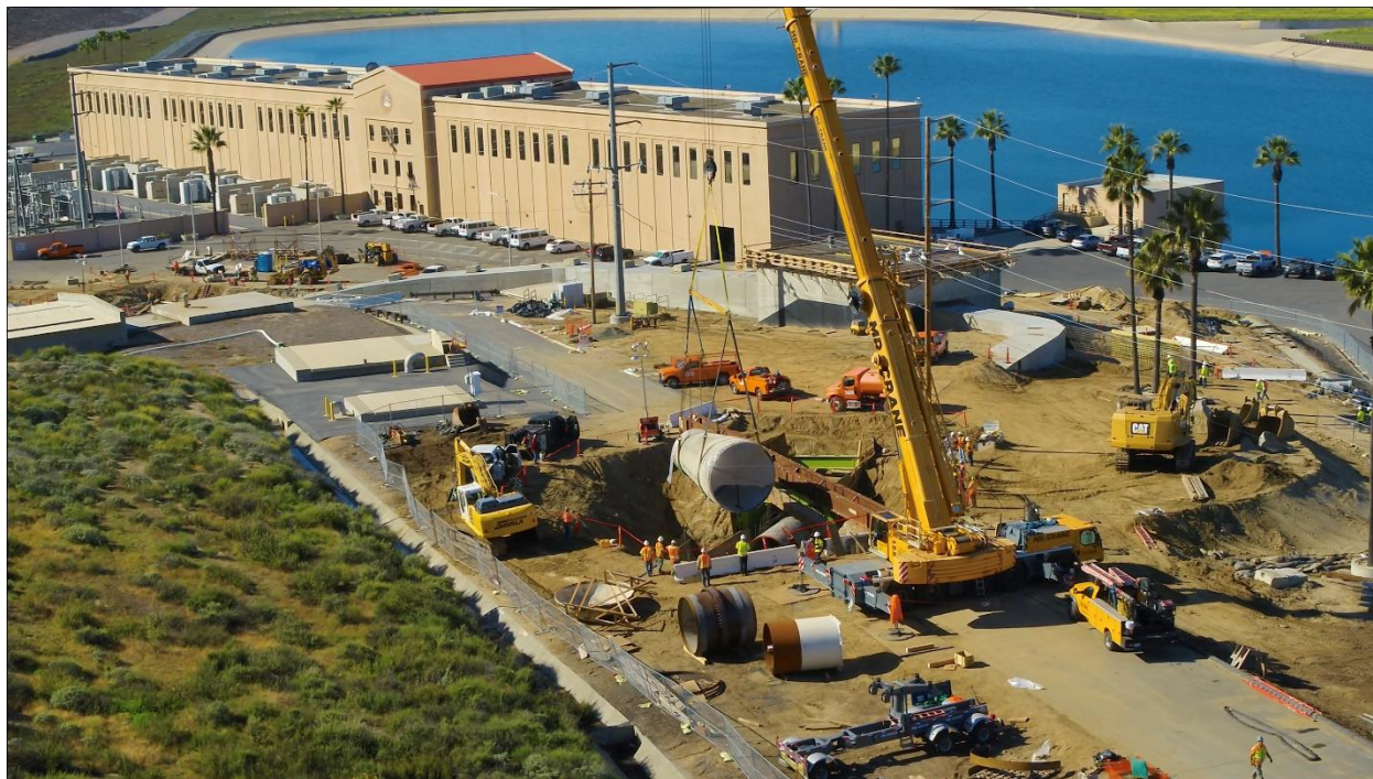
Contractor using crane to lift bypass tie-in pipeline
