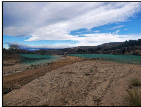
Hydroseed Application for the Foothill Feeder Exposed Barrel Repair Project
