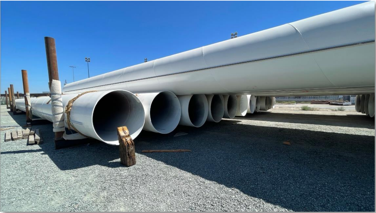
Figure 32 – Steel Pipe Piles at DWR Stockton Yard
