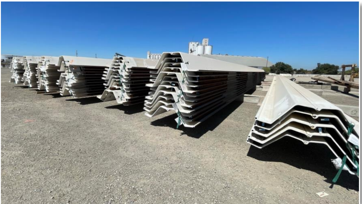
Figure 31 – Sheet Pile at DWR Stockton Yard
