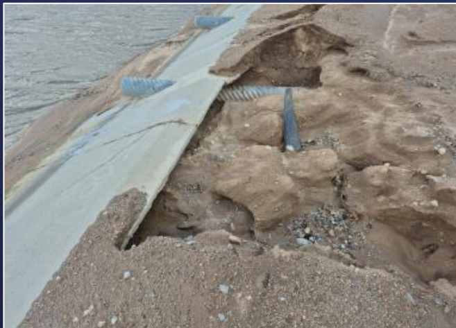
Buckled and undercut panels along East Branch
