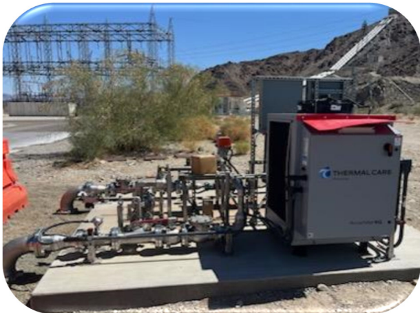
Eagle Mountain Domestic Water Chiller (Start-up and commissioning are in progress)
