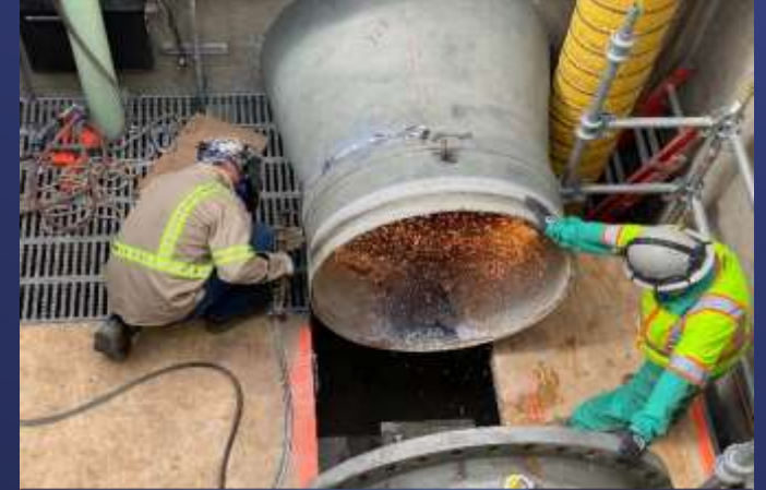
Pipe Spool Removal
