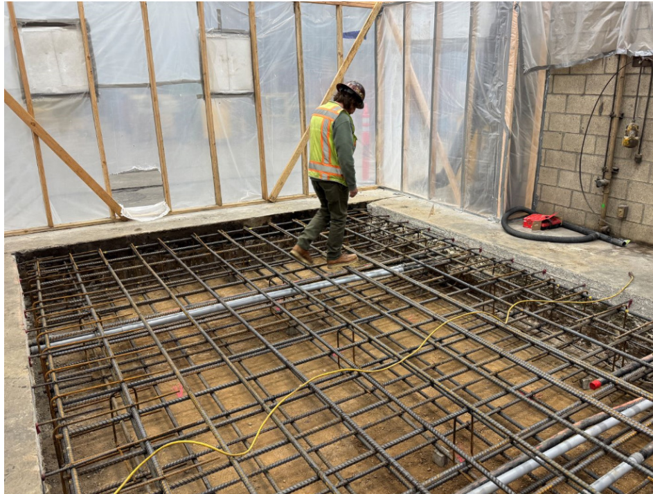
La Verne Shops Improvements — Inspecting Reinforcement for the Vertical Saw Foundation
