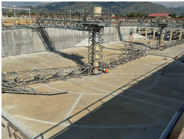
Existing equipment removed from the sedimentation basins at the Weymouth plant
