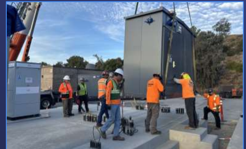
Jensen Battery Energy Storage System (BESS) Installation
