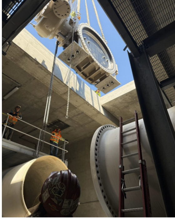
Wadsworth Bypass — Installing the 84-inch Butterfly Valve
