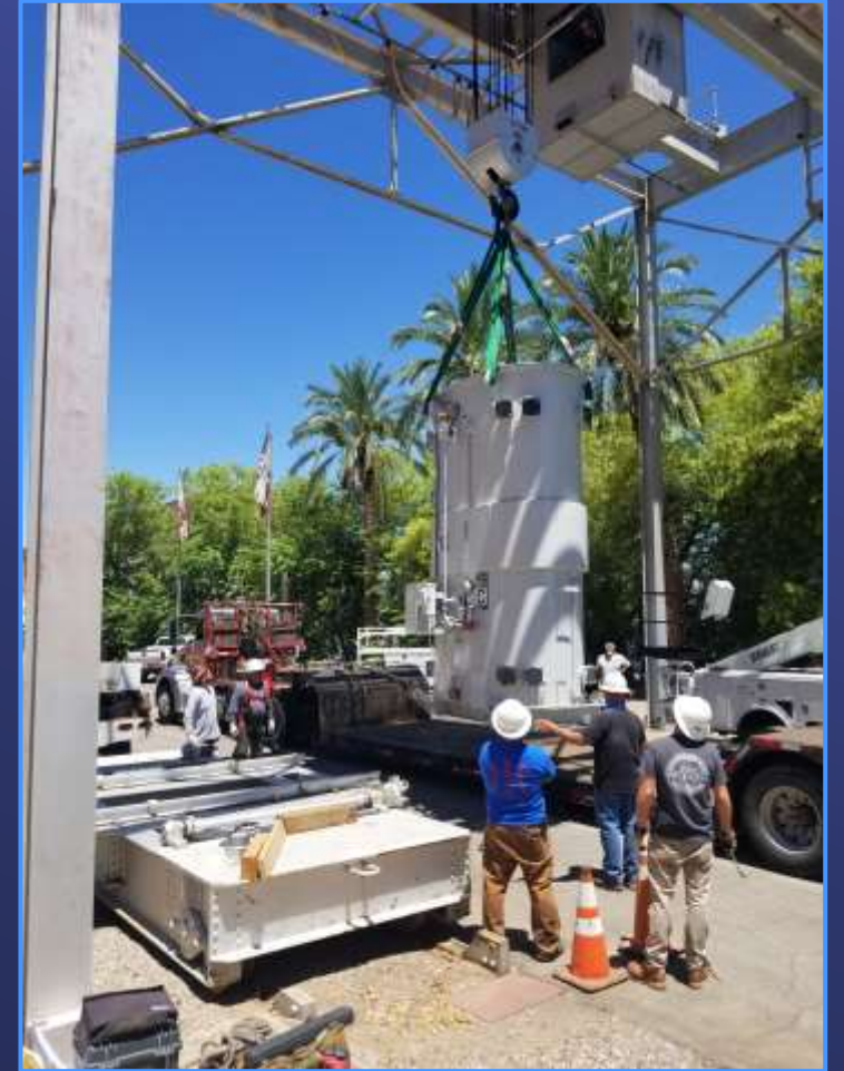
Staff Installing Refurbished Intake 2C Transformer Unit (Removed 10/19, Installed 6/20, Energized 2/21)
