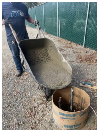
Staff pouring concrete base (left) and installing new light fixture (right)
