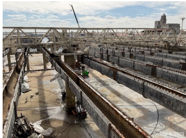
Existing equipment removed from the sedimentation basins at the Weymouth plant
