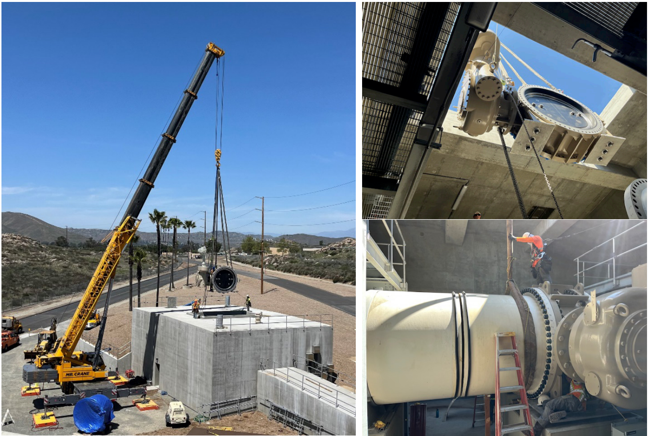
Staff lowering an 84-in butterfly valve into position for the Wadsworth Bypass
