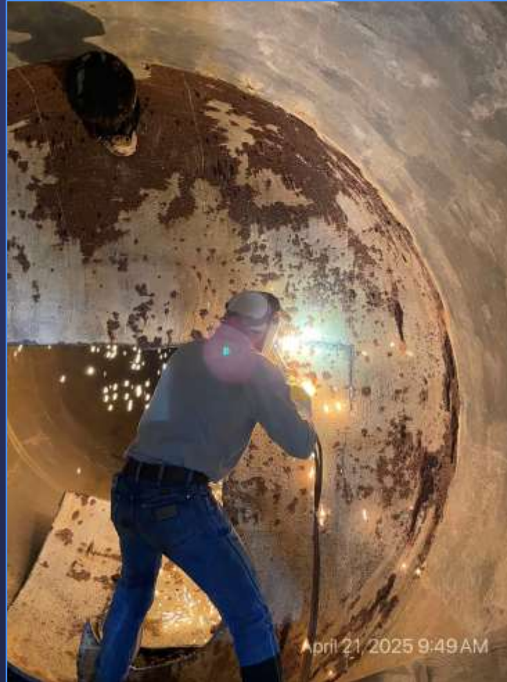
Welder Cutting Bulkhead
