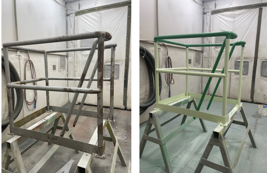
Gene Unit 1 discharge valve pit handrail before (left) and after (right) coating
