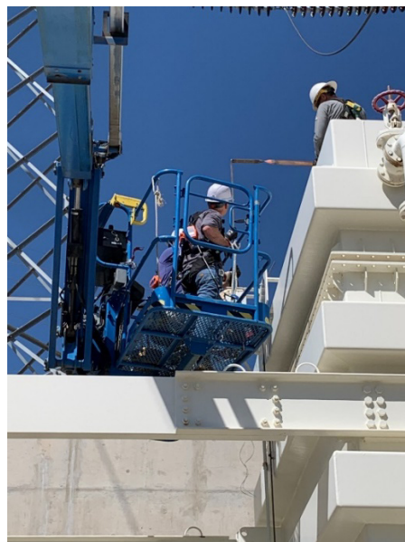
Staff installing spare transformer neutral CT (left) and fabricating bus for neutral CT connection (right) at Hinds pumping plant
