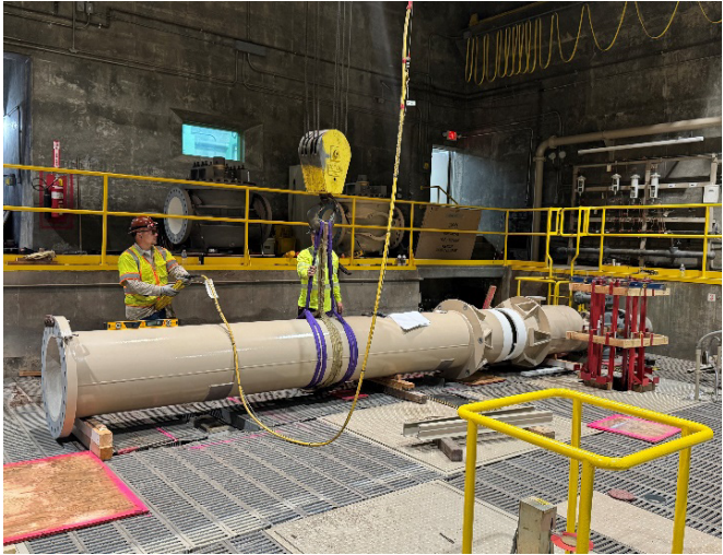
Staff hoisting pipe section into place at the Oak Street PCS
