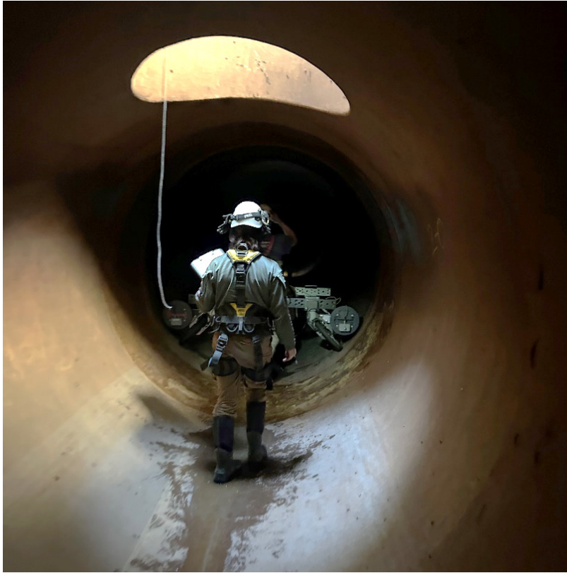
Yorba Linda Feeder PCCP Electromagnetic Inspection
