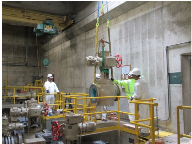
Staff installing a new 12-inch lubricated plug valve (left) and hoisting a refurbished 16-inch hydraulic globe valve for installation (right) at Covina PCS
