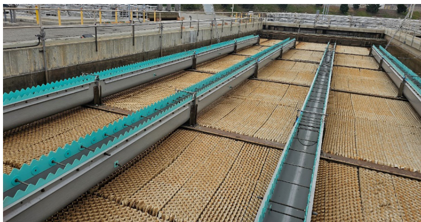
Newly refurbished launder troughs at Skinner Washwater Reclamation Plant
