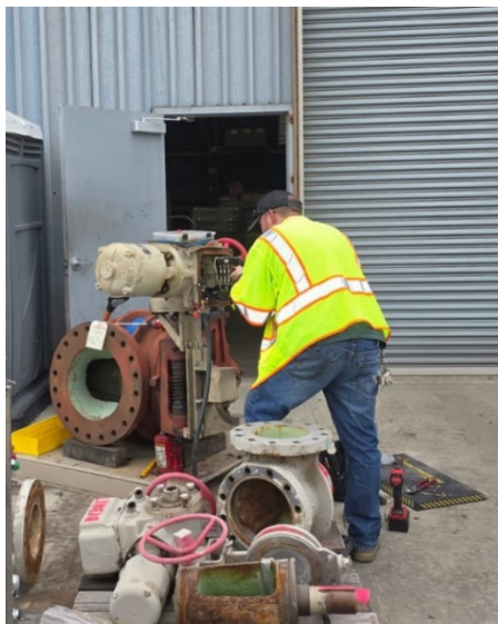
Staff setting valve limits (left) and rewiring and testing valves (right) at Covina PCS
