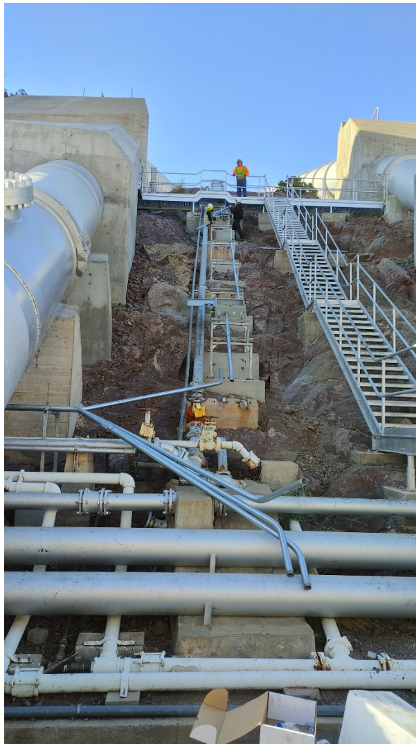
Contractor installing electrical conduits at Intake Pumping Plant
