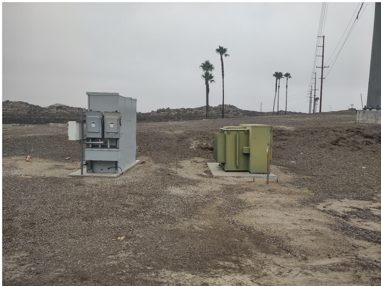
Wadsworth Pumping Plant Bypass Pipeline project site [Looking northward toward the plant entrance gate showing electrical switch gear, which will be relocated]
