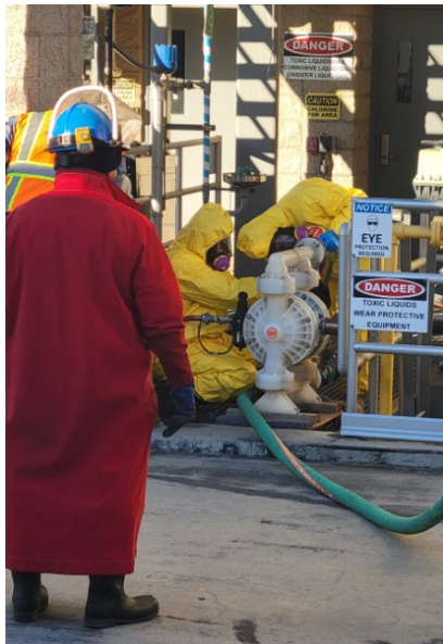
Vendors hooking up pump to recover caustic solution (left) and equipment and materials staged to expedite repairs (right)
