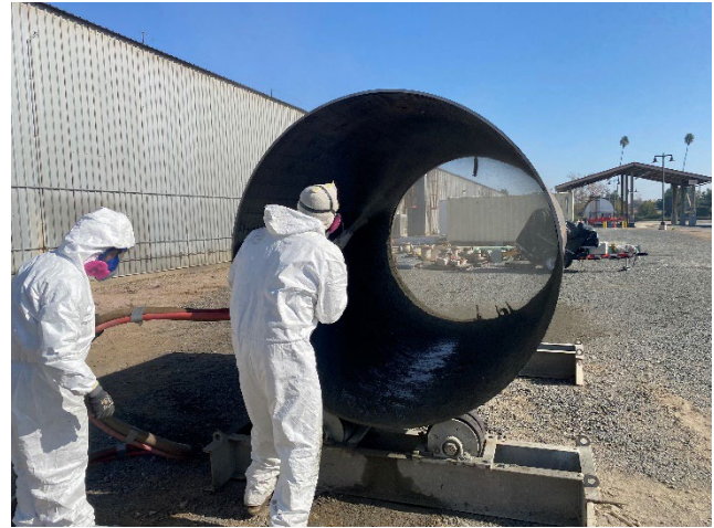
Staff mixing mortar and loading pump (left) and applying mortar to pipe interior (right)
