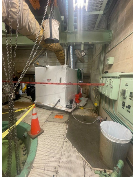
Containment for blasting and coating of discharge valve
