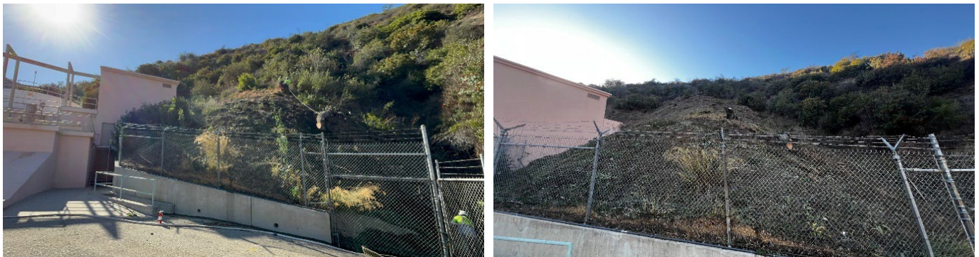
Completed clearing of brush on hillside at Sepulveda PCS
