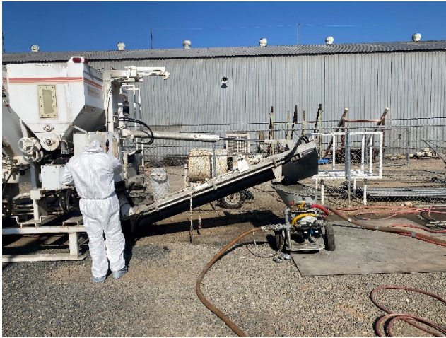
Staff mixing mortar and loading pump (left) and applying mortar to pipe interior (right)
