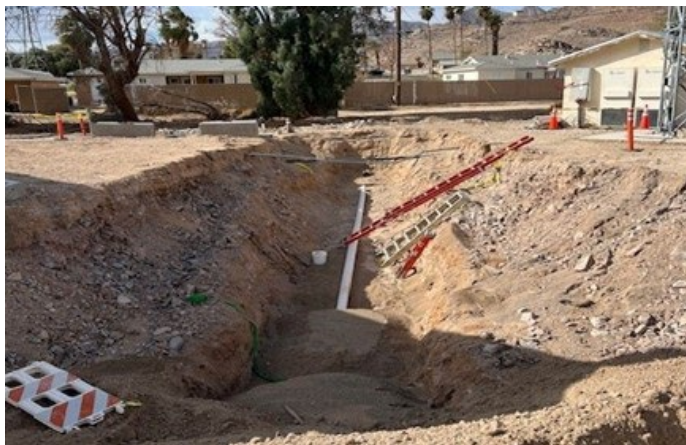
Iron Mountain sewer line replacement
