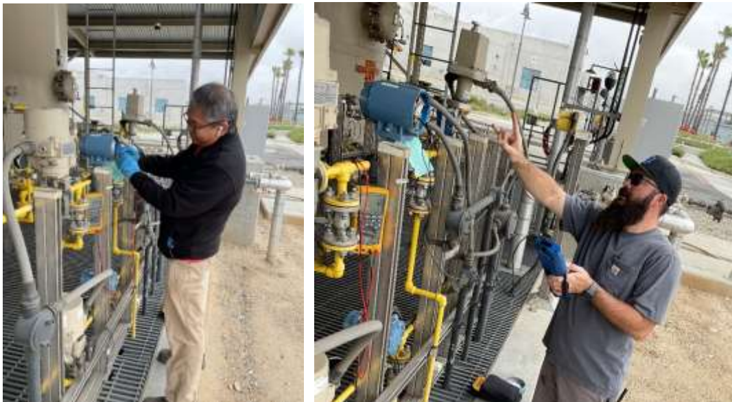
Staff installing and verifying ammonia flow meters at the Weymouth plant
