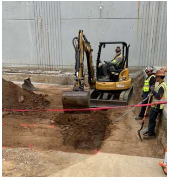
La Verne Shops Building Completion, Stage 4, Equipment pad excavation
