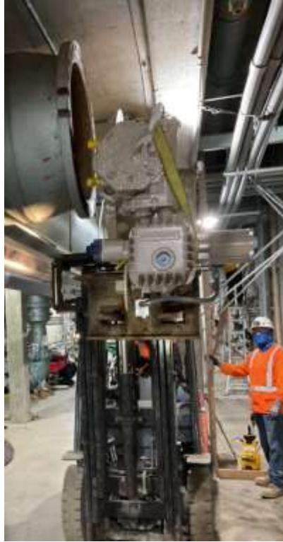
Weymouth Basins 5–8 and Filter Building No. 2 Rehabilitation Backwash Valve Installation
