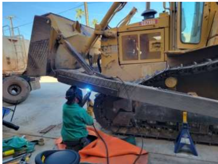
Staff welding a dozer arm to repair wear from recent project usage at a Desert facility
