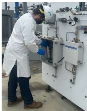
Staff collecting microbial samples following secondary membrane bioreactor treatment at the PWSC demonstration plant
