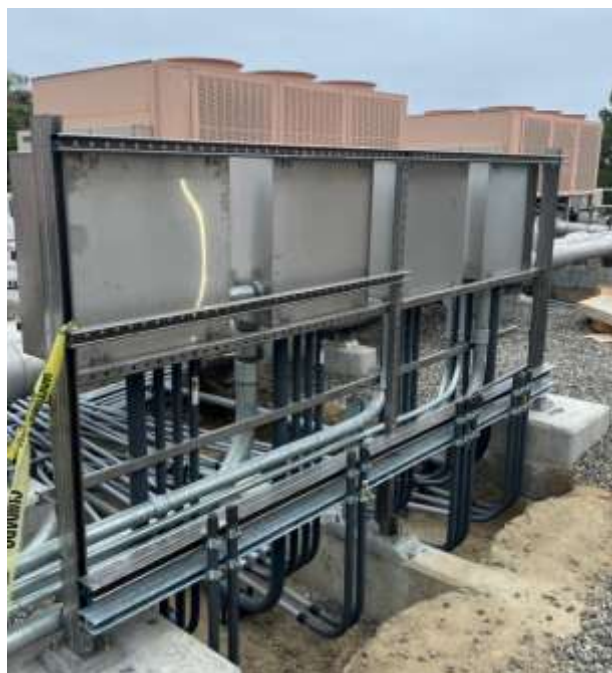
Figure 10C-88 Pump Station Chillers Replacement Electrical Conduit Installation
