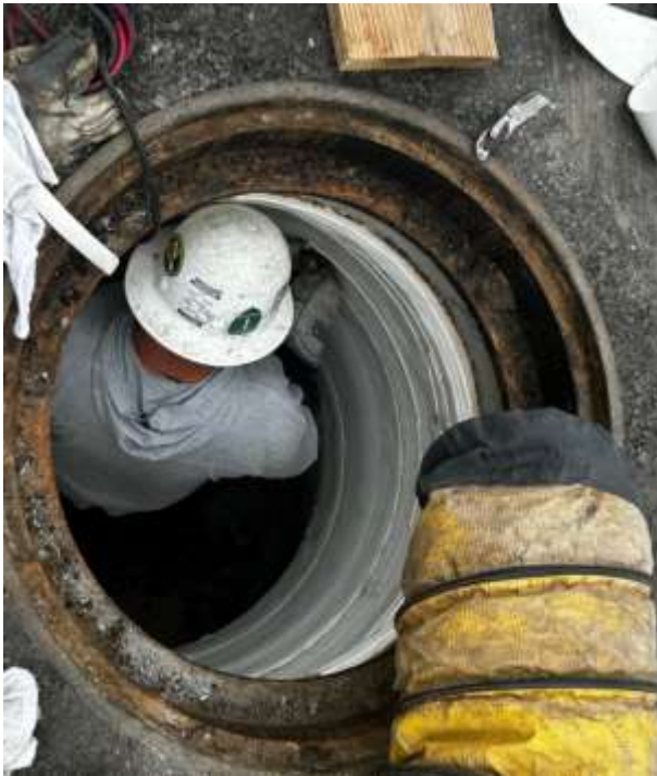
Lake Mathews Wastewater Replacement Installation of containment lining inside manhole
