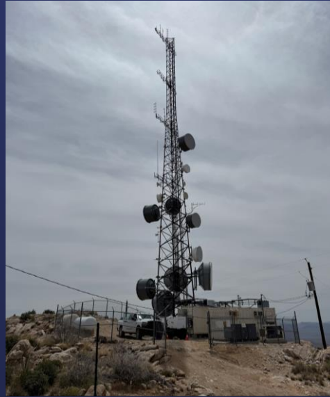
Completed Installation of 6 Microwave Antenna at Christmas Tree Pass
