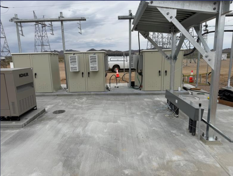
Installation of MFE Outdoor Enclosures and Propane Generator at Camino Sub Station
