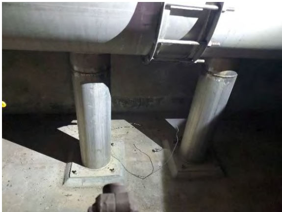
Supports to be cut (left), and valve and actuator to be replaced (right)
