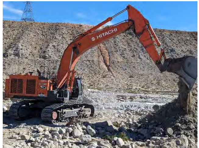
Equipment pushing material along the CRA (left) and reinforcing protective berms (right)
