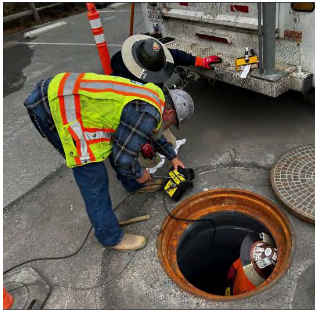
Lake Mathews Wastewater Replacement—Testing manhole coating
