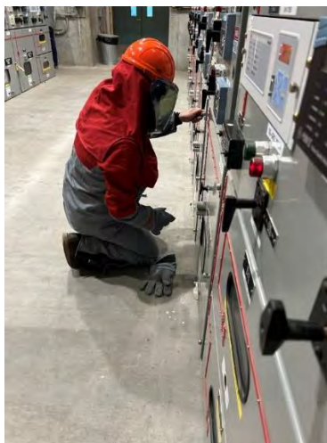
Staff performing high-voltage switching to safely isolate electrical equipment for maintenance
