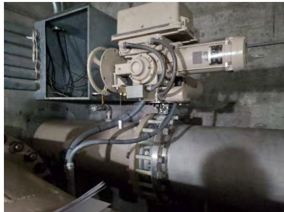
Supports to be cut (left), and valve and actuator to be replaced (right)
