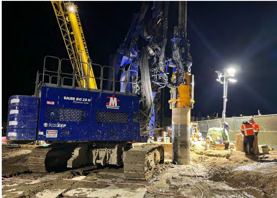
Perris Valley Pipeline —Drilling secant piles for Shaft No. 3
