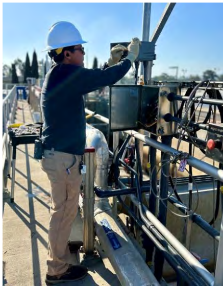
Staff connect a new nitrate probe to assess denitrification in the anoxic tank at the demonstration plant
