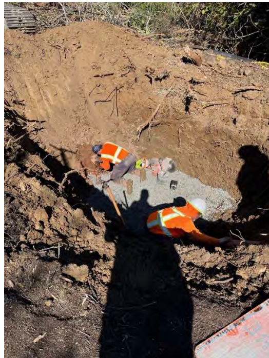
Damaged sewer line at Diemer plant
