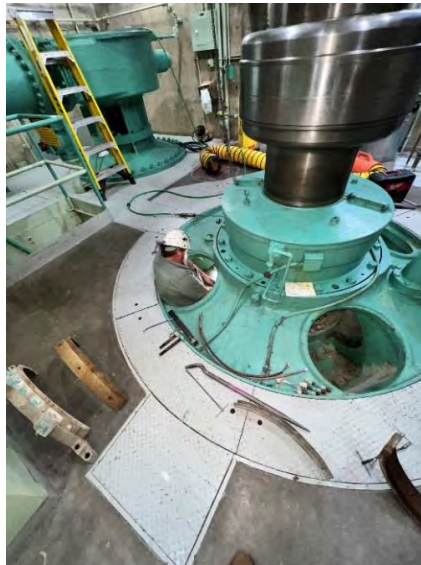
Staff cleaning and replacing pump bowl packing at Eagle Mountain pumping plant
