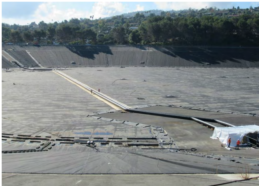
Temporary bypass for the Palos Verdes Feeder at Palos Verdes Reservoir
