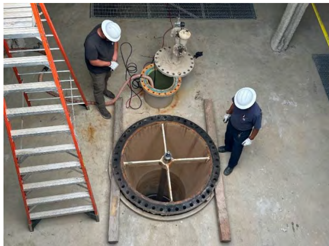
Staff preparing to remove sleeve valve for refurbishment at PC-1
