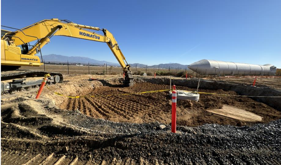
Perris Valley Pipeline Tunnels—Backfilling and compacting at tunnel shaft site
