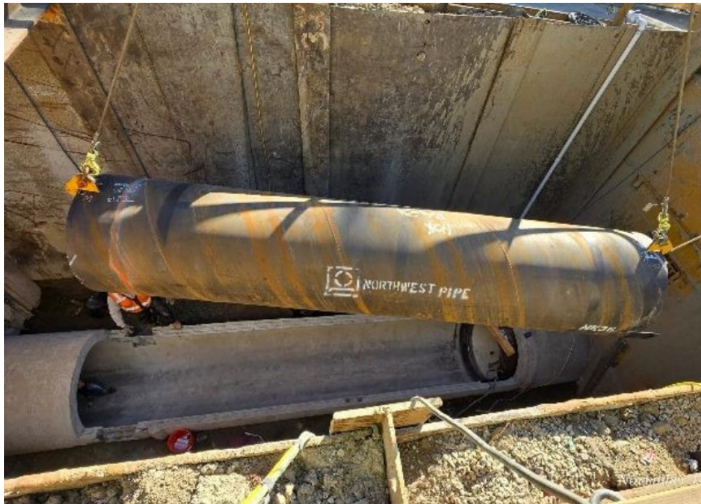
Allen-McColloch Pipeline (AMP) Urgent Relining—Steel Liner Pipe Installation
