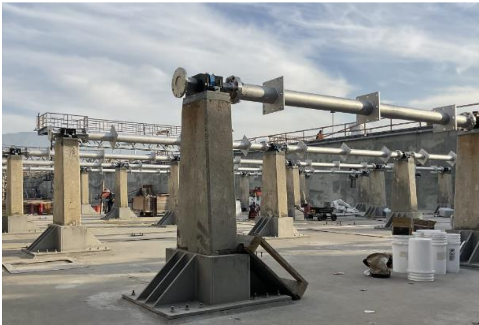
Weymouth Basins 5–8 and Filter Building No. 2 Rehabilitation— Basin 6 Flocculator Shaft Installation
