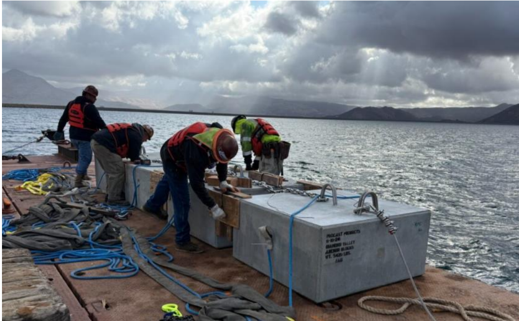
Diamond Valley Lake Wave Attenuator—Preparing Concrete Anchor Blocks for Installation
