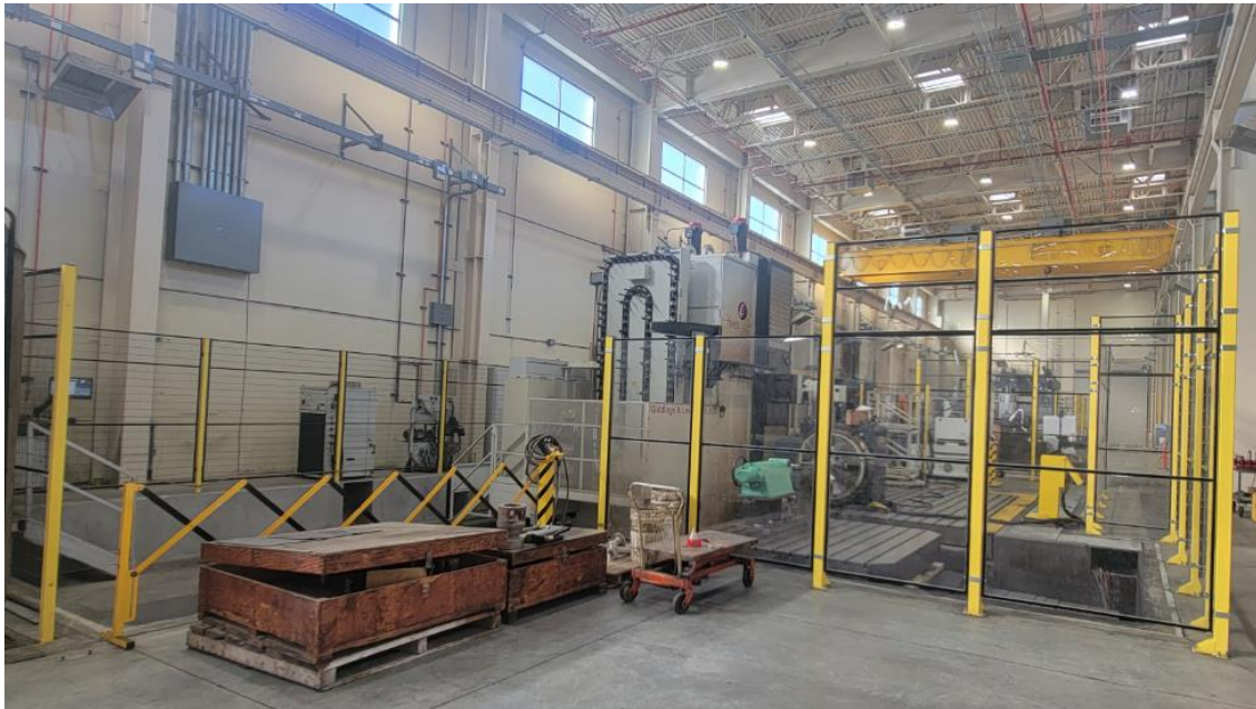
La Verne Shops Improvements—Safety fencing installed around existing Horizontal Boring Mill
