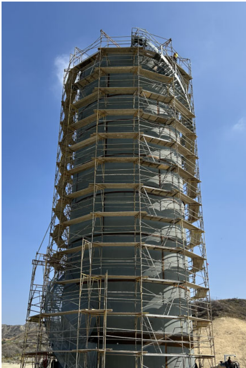
Inland Feeder-Badlands Tunnel Surge Protection –Scaffold Install for Tank Coaters
