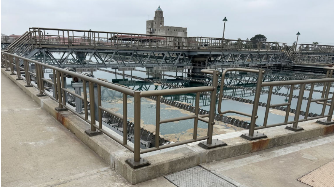
Weymouth Basins 5–8 and Filter Building No. 2 Rehabilitation — New Handrail Base Plates at Basin 6
