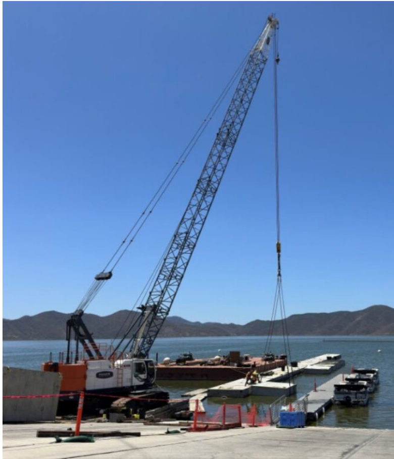
DVL Wave Attenuator Replacement — Setting Concrete Modules in the Water
