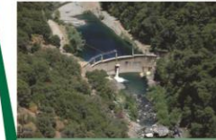
▲ Our House Dam
