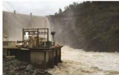
⚡ Narrows II Powerhouse
