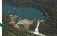
▲ New Bullards Bar Dam
