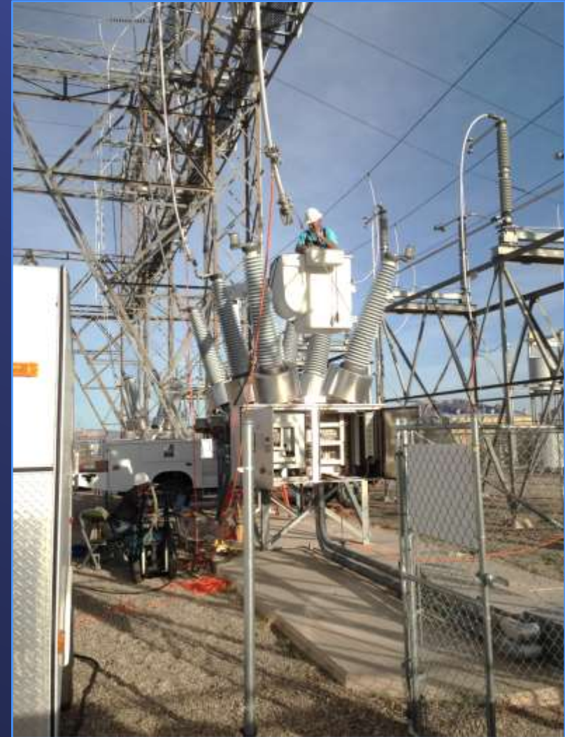
Switchyard Equipment Testing
