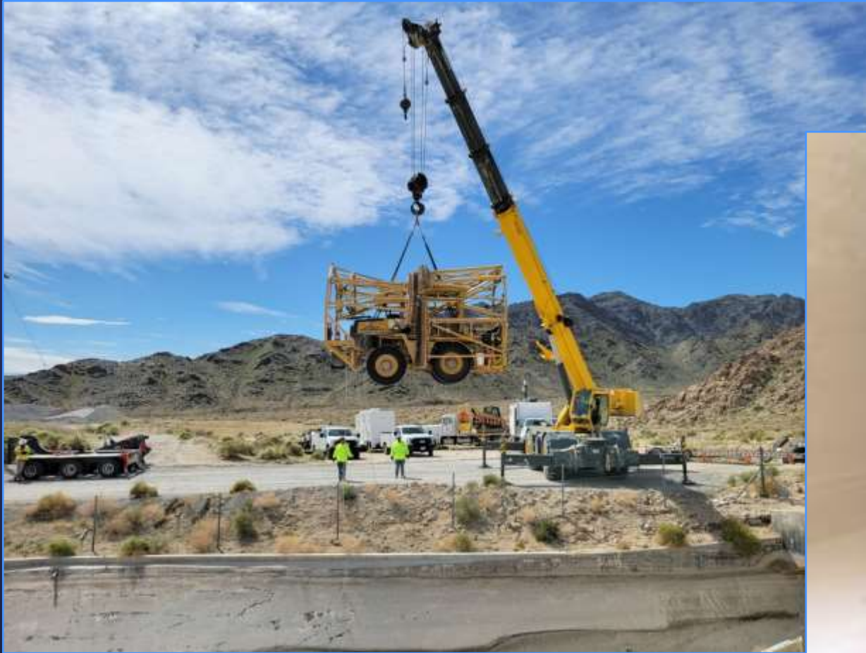
Tunnel Cleaning Machine Setup
