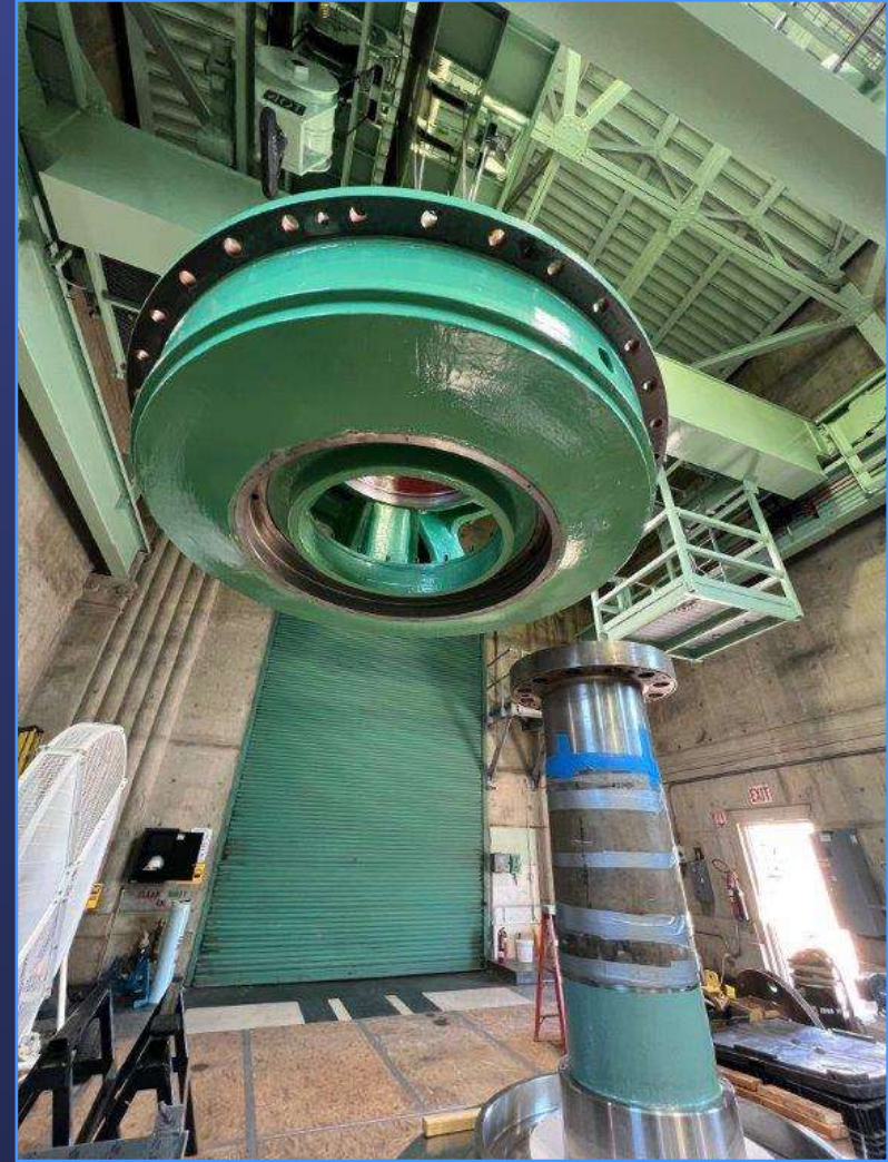
Unstacking of Pump Unit
