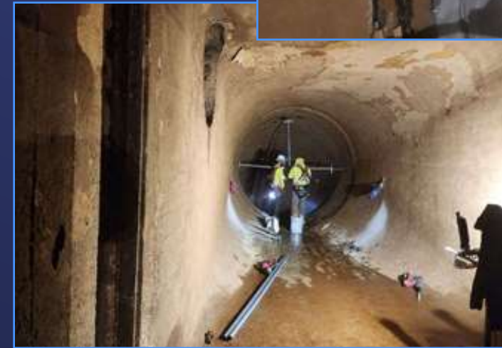
Eagle Mountain Transition Joint Repairs
