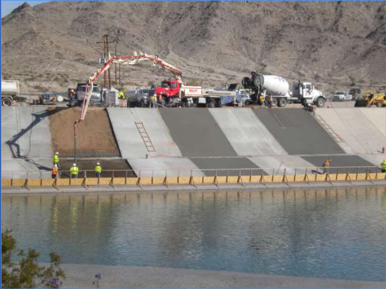
Iron Mtn. Reservoir & Canal Liner Replacement $4.7M (Completed: 2019)
