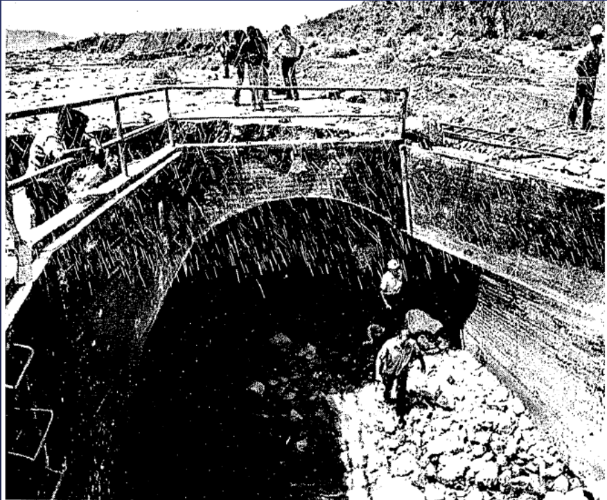
SHUT DOWN --Damaged Colorado River Aqueduct structure east of Desert Hot Springs after a 10-foot wall of mud and boulders swept away the hatch and clogged system with debris. Times photo by Andy Hayt
