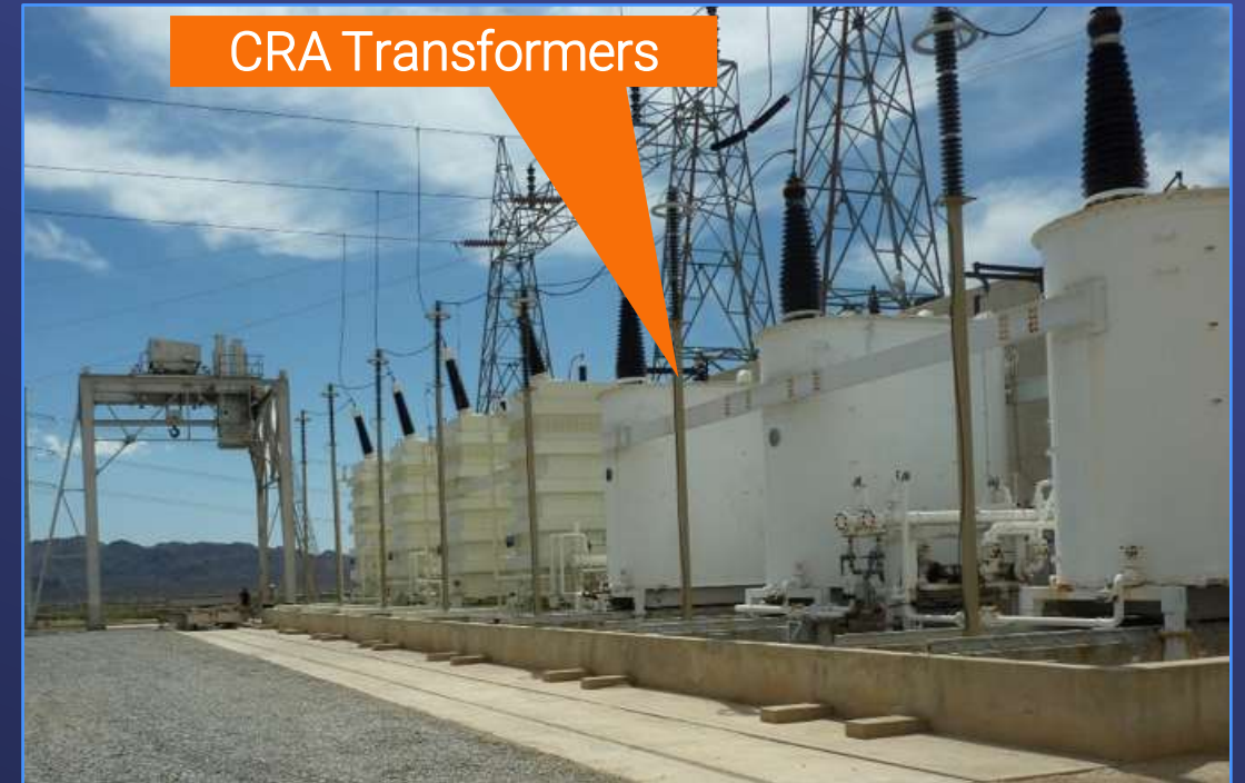
CRA Transformers Replacement (Planned design completion: 2025) $120M
