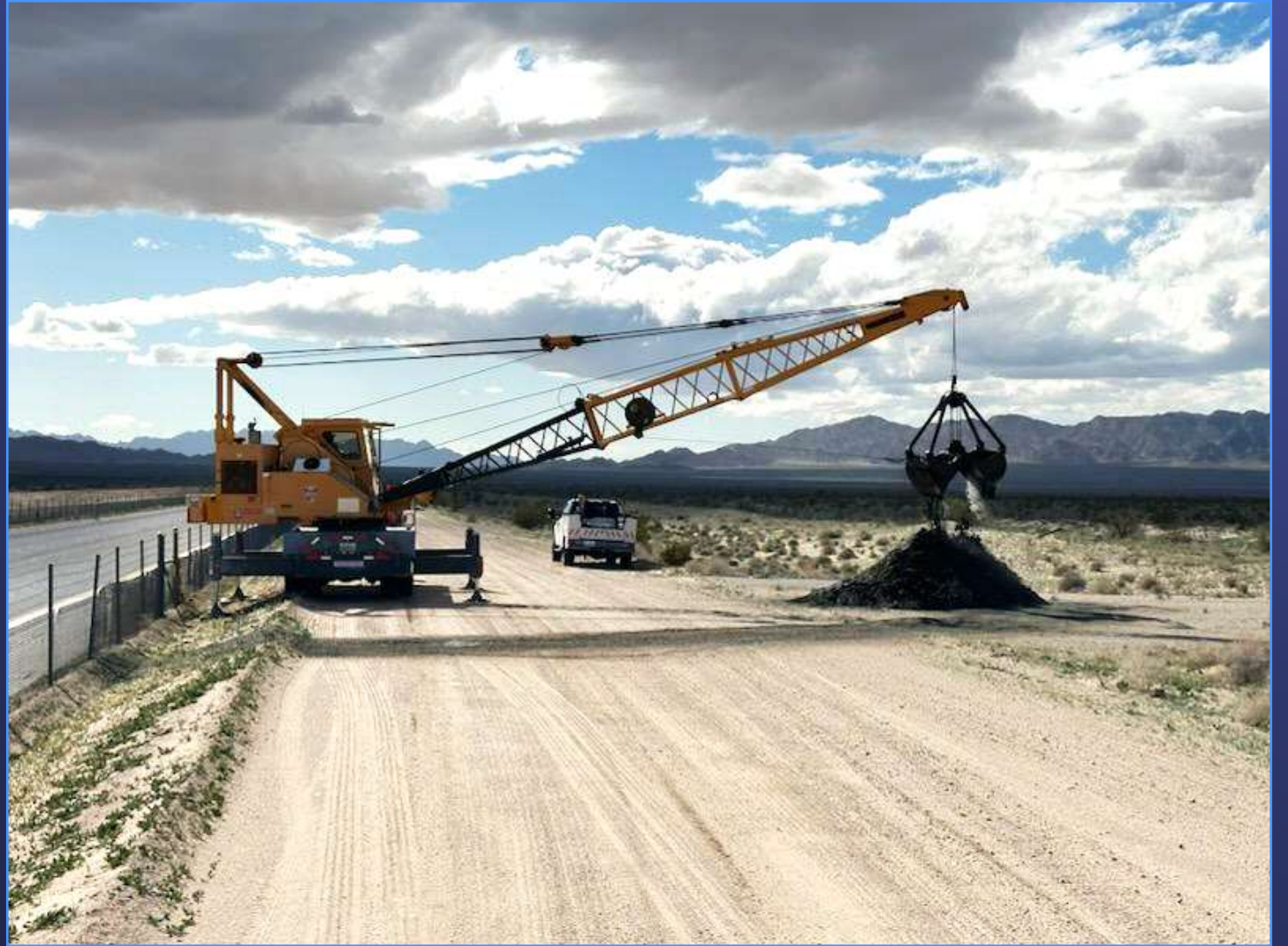
Canal Sand Removal
