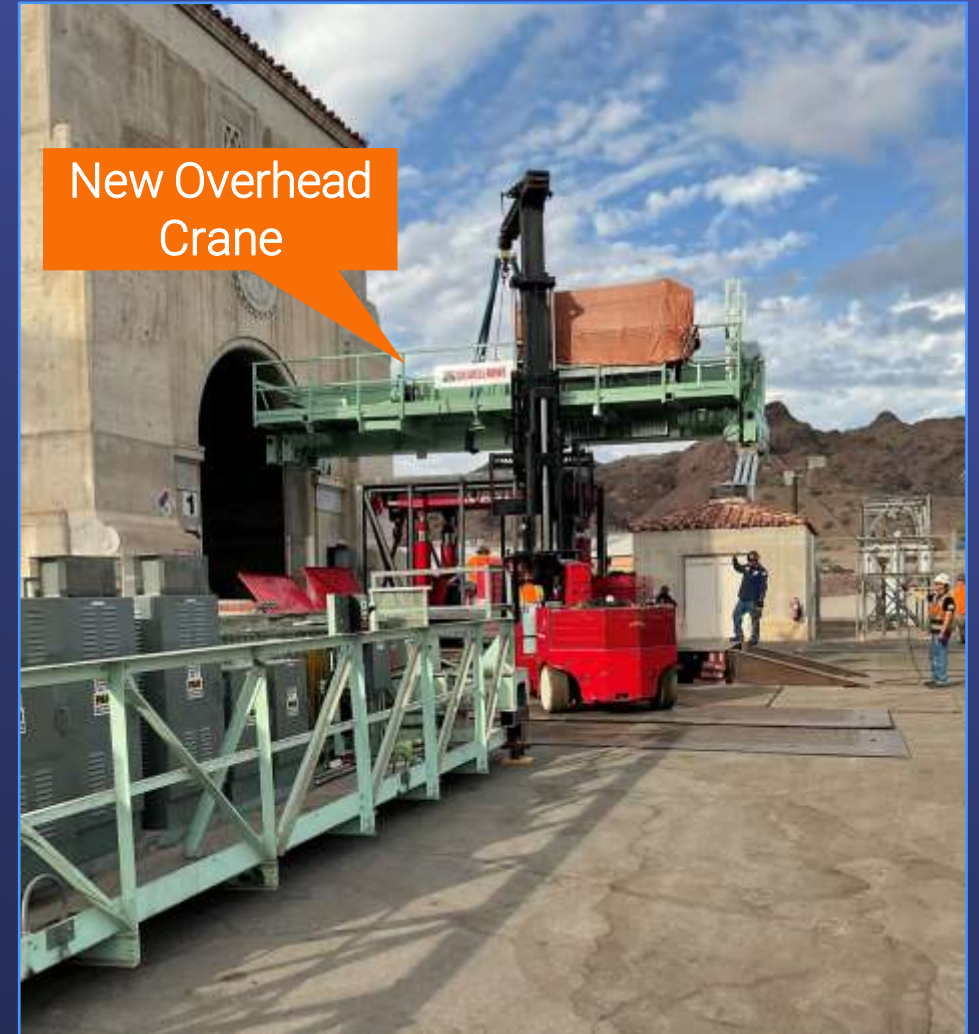
CRA Overhead Cranes Replacement (Planned completion: 2024) $13.4M
