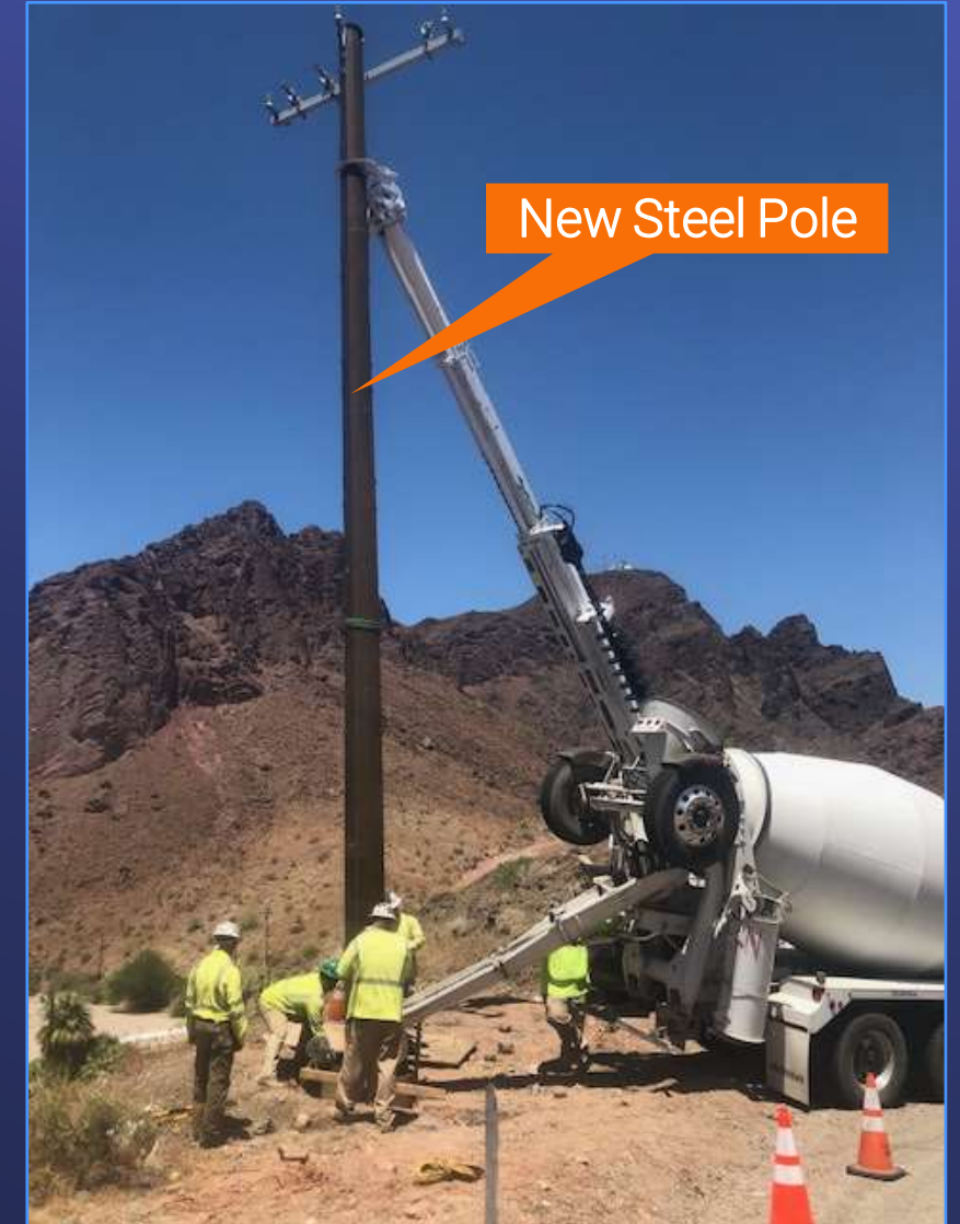
Intake 2.4kV Power Line Upgrades $5.5M (Completed: 2018)
