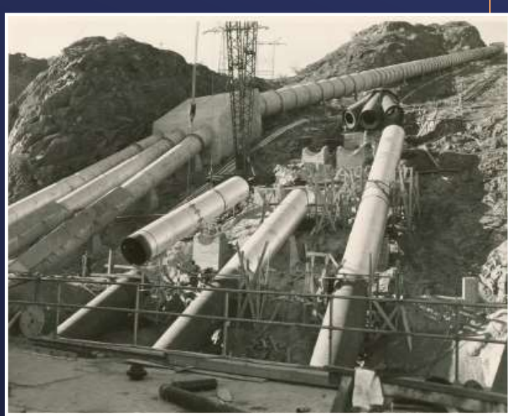
Intake Pumping Plant 1955
