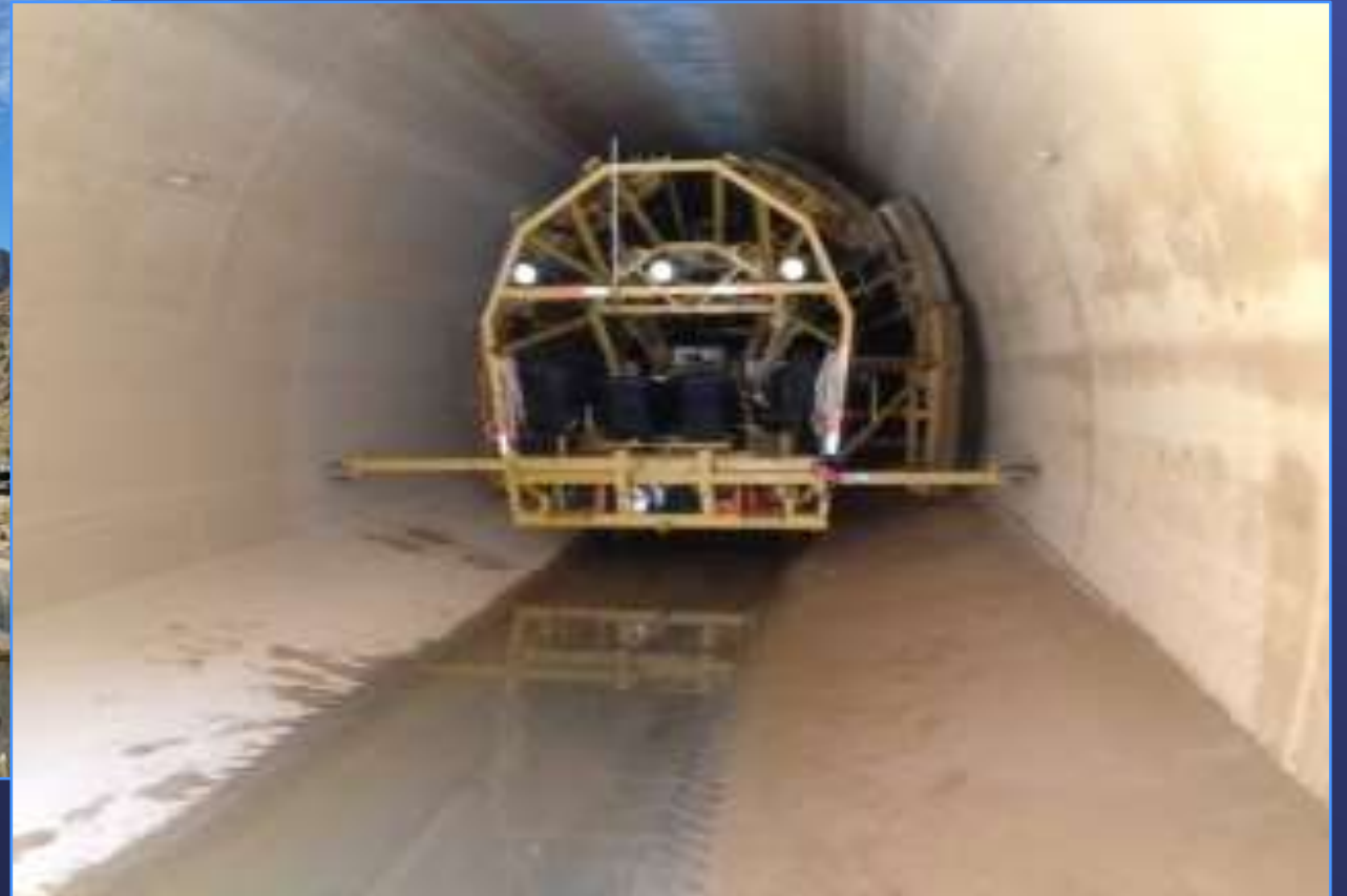
Tunnel Cleaning Machine at Work
