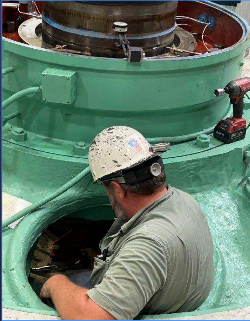
Iron Mtn PP Pump Unit Maintenance
