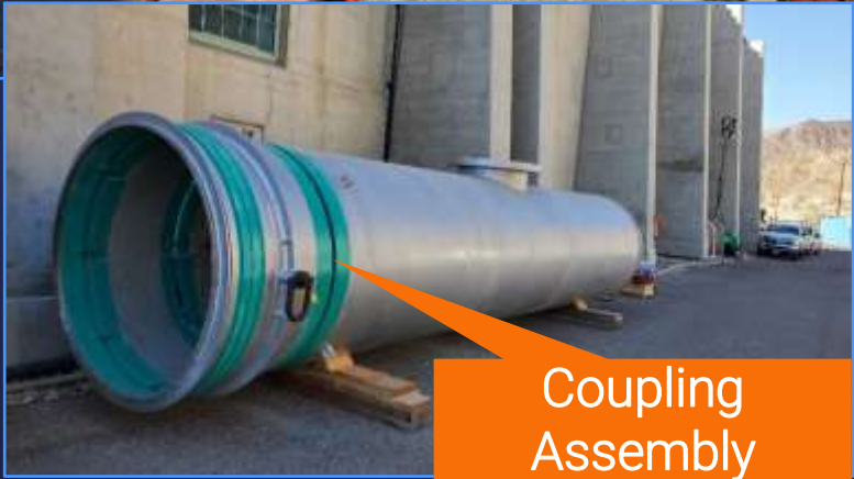
Discharge Line Isolation Couplings $32.9M (Completed: 2021)
